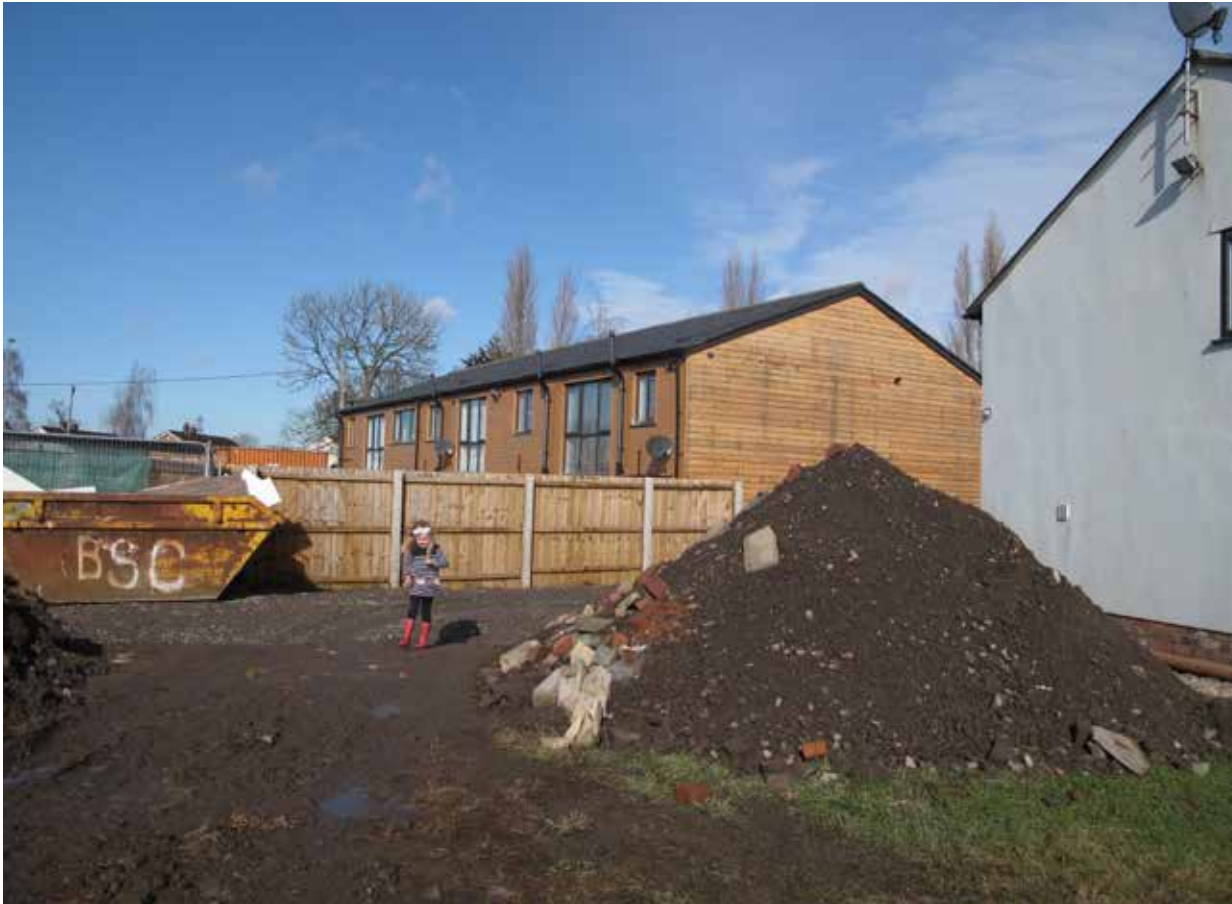
Photograph towards the North of the site showing the neighbouring properties.
