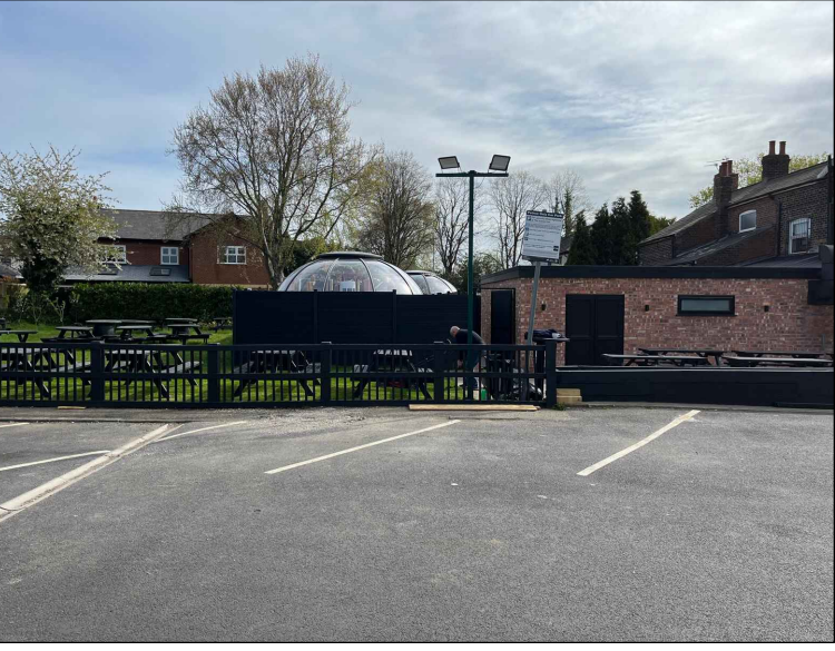
Terrace view from Car Park
