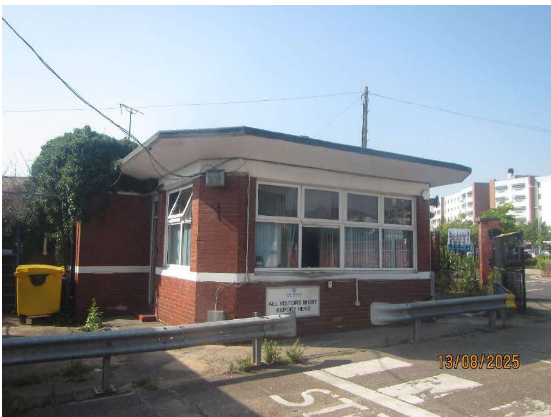
Photograph 10. The eastern and southern aspects of Building 4.
