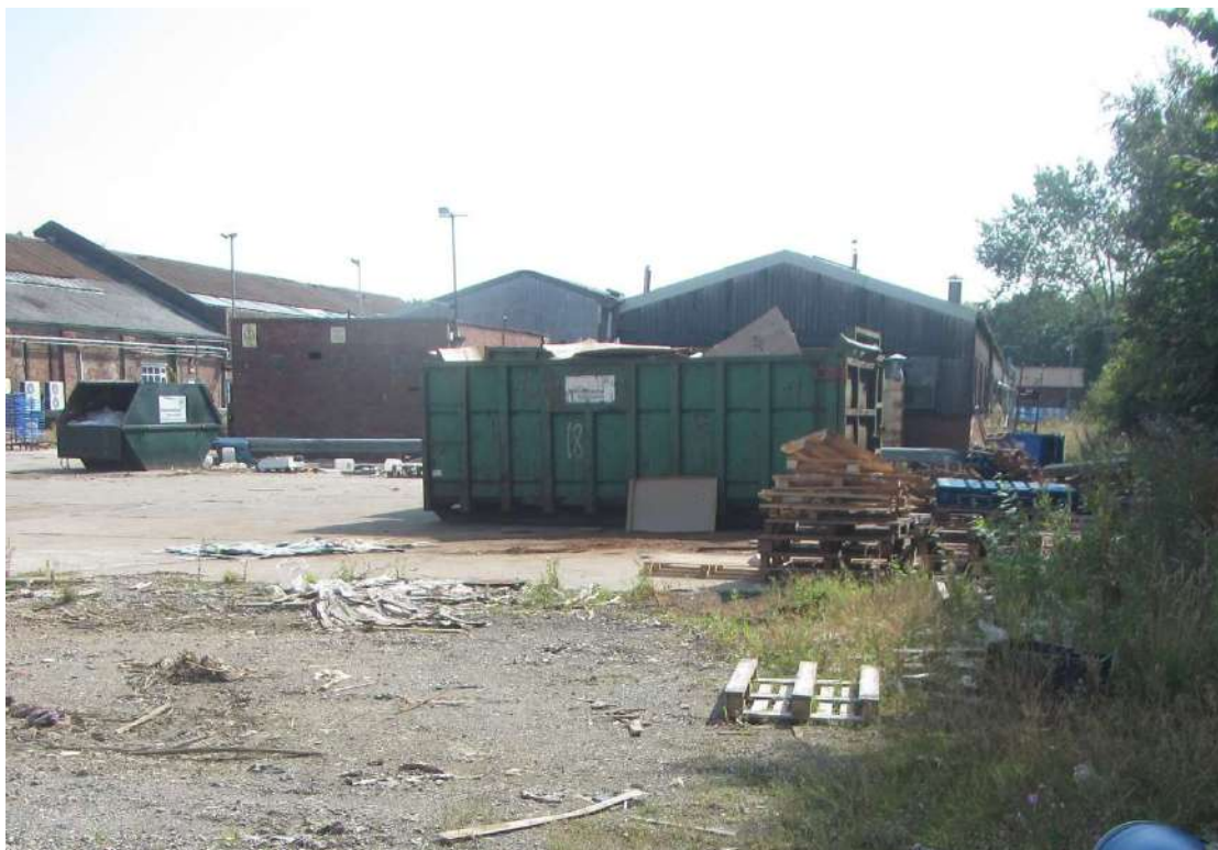
Photograph 8. The western aspect of Building 3.
