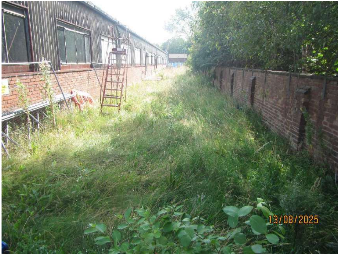
Photograph 9. The southern aspect of Building 3.
