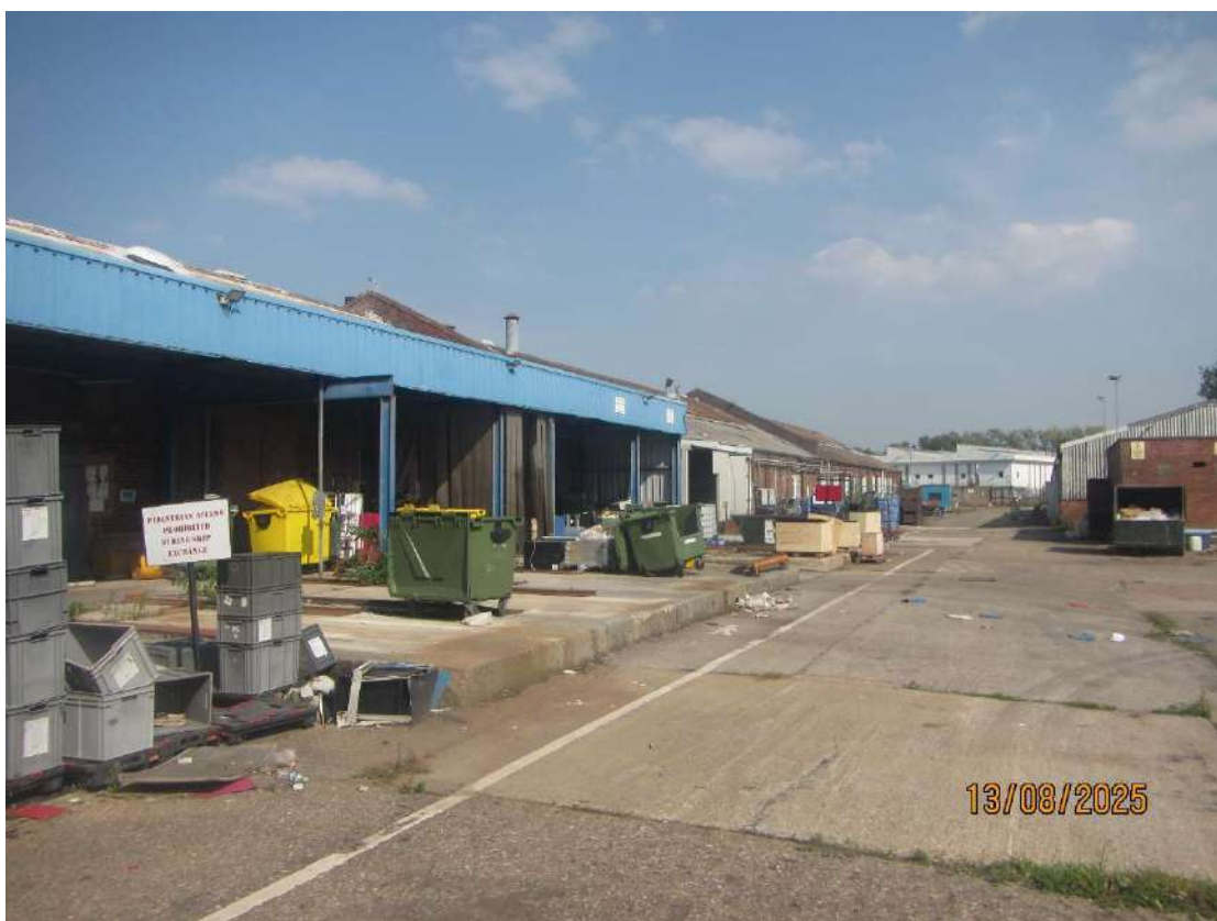
Photograph 4. The southern aspect of Building 1.
