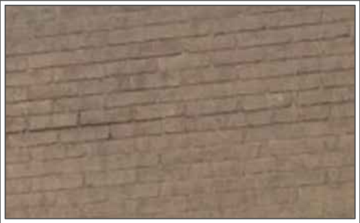
Existing brickwork to be retained and cleaned
