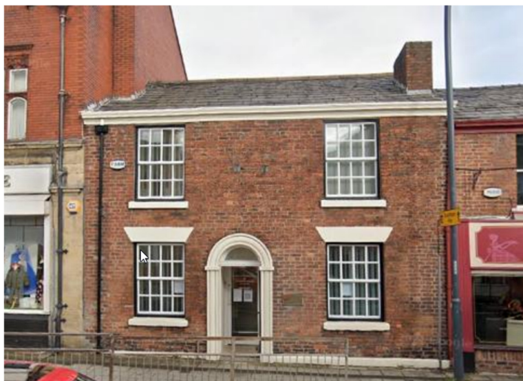
37 High Street, unaffected by the proposed work at 40 High Street
