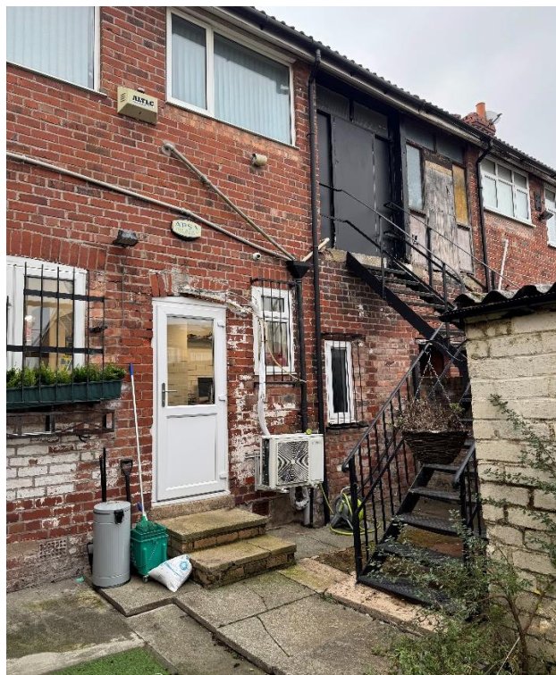
Photo: Rear of shop with predominantly concrete hardstanding and small area of astro turf.
