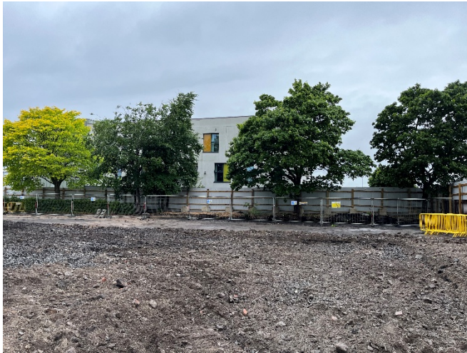
Tree protection zone, with warning signage
