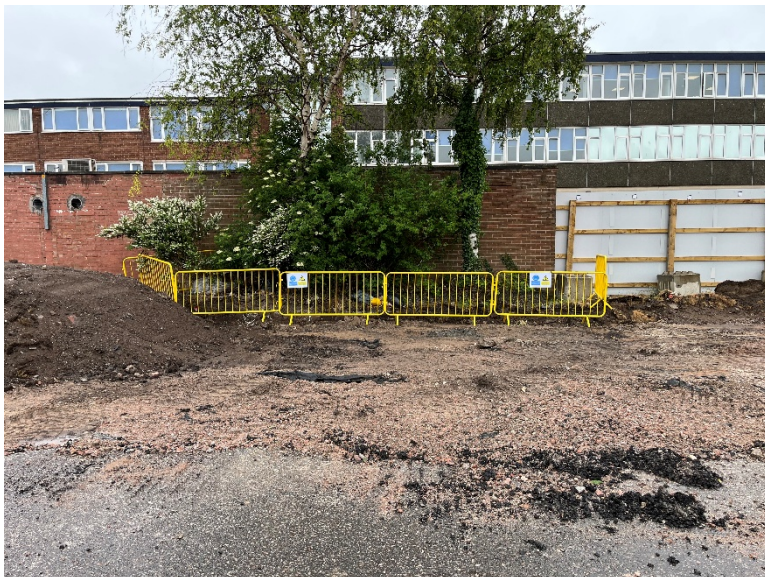
Tree protection zone, with warning signage
