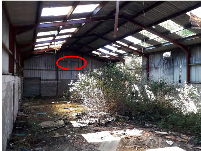
Plate 4: Internal view of Building 2 (pigeons were nesting on the metal framework at the end)
