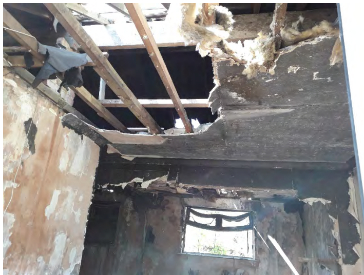
Plate 3a, 3b: Internal views of Building 1
