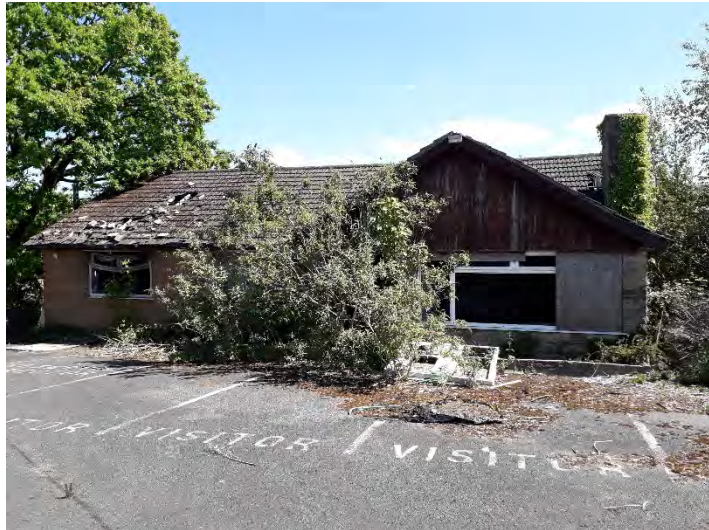
Plate 1a, 1b: External views of Building 1
