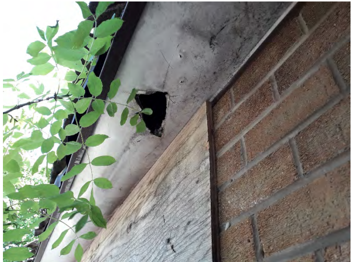
Plate 2a, 2b: External potential roost features of Building 1
