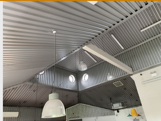
Photograph 2: Internal metal ceilings within B1.
