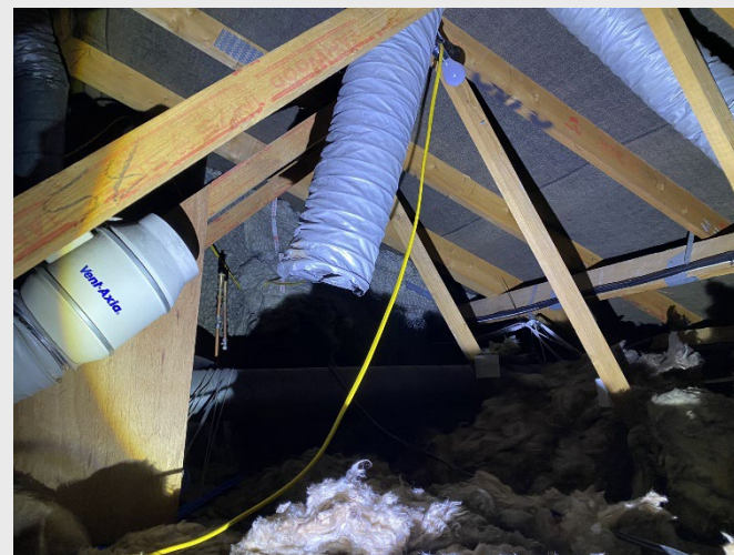
Photograph 4: Example of loft space within B1 with wooden ceiling beams.
