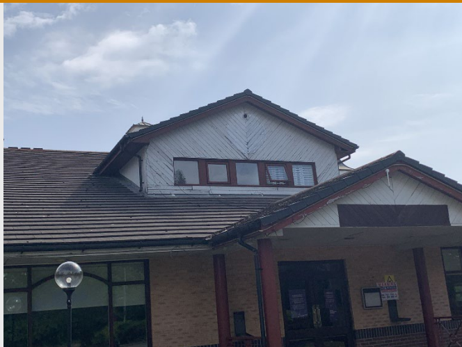
Photograph 1: Western aspect view of Building B1.
