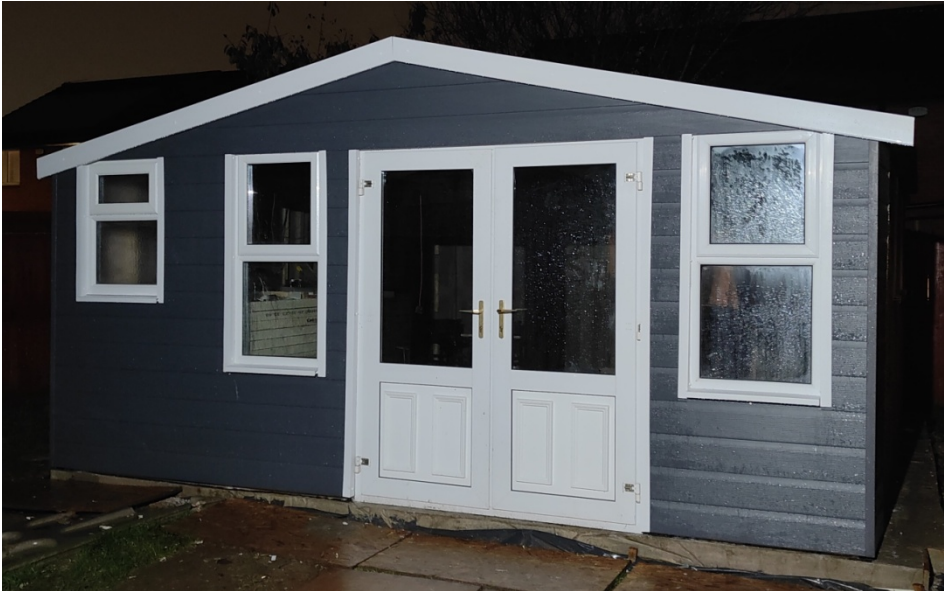
Garden Room Current progress photograph.
