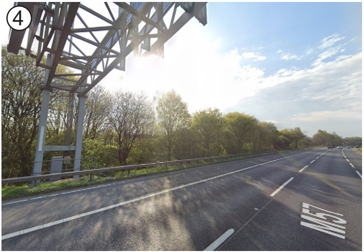
Viewpoint 4 View along the M57 Motorway, looking south east towards the development site.
