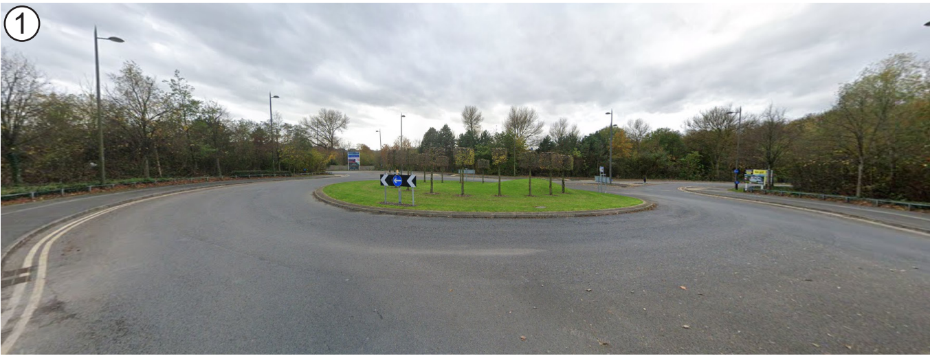
Viewpoint 1 View of the Carr Lane/ Prescott Park Way roundabout.
