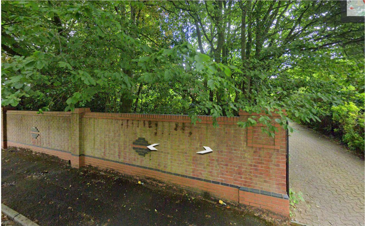
Neighbouring Property boundary wall
