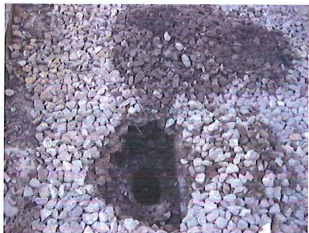
HDP01 excavation (duct visible to right of image)
