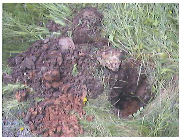
Arisings and excavation HDP06
