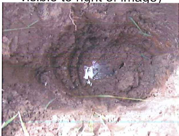
HDP02 excavation (black duct visible)
