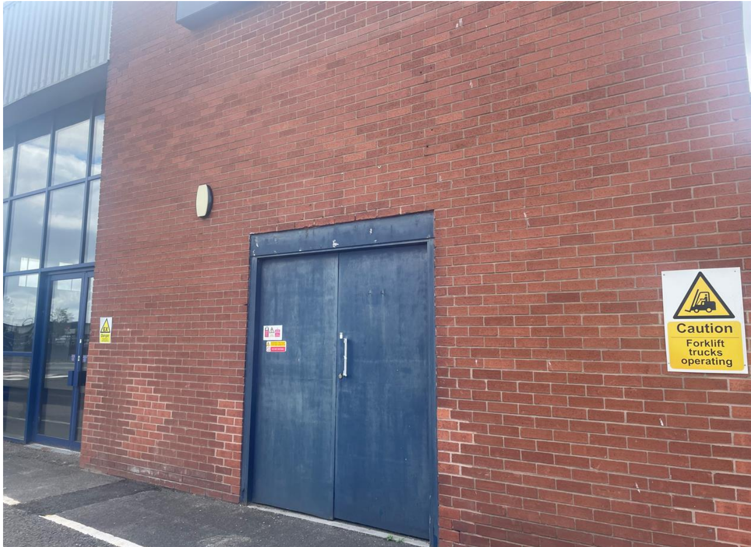
Photo 12: Access point to eastern side of building.
