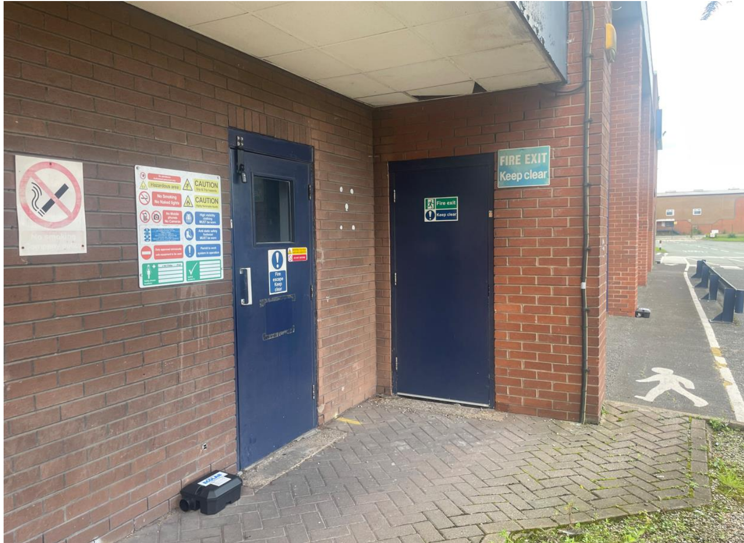
Photo 15: Access points into the eastern side of the building, outside an office area.
