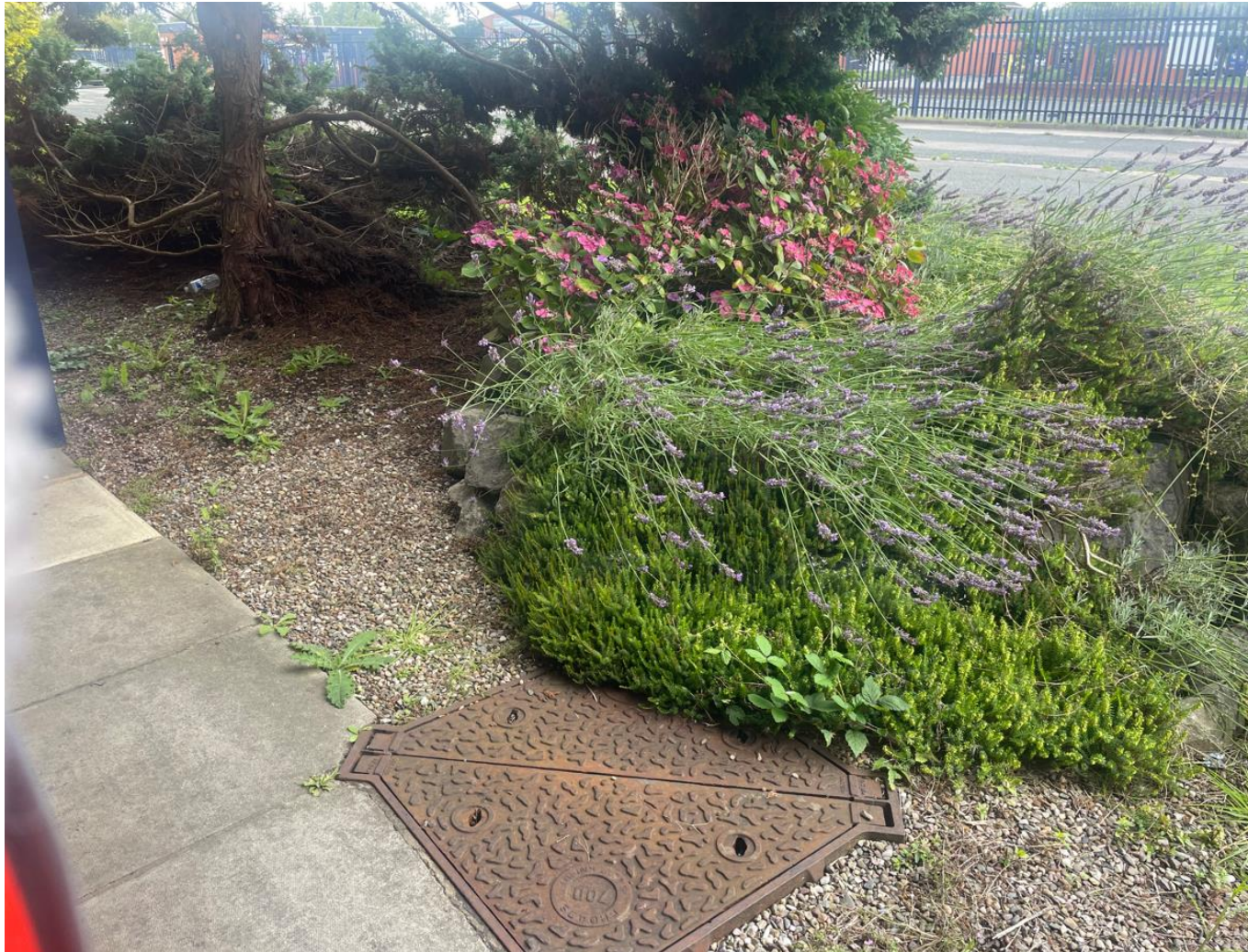
Photo 17: Soft landscaping area, including small trees and bushes, outside the front of the eastern side of the building. A drain cover is present.
