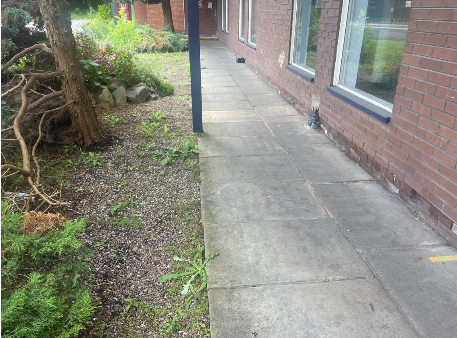
Photo 18: Soft landscaping to the left, including small tree. A concrete slab pathway runs along eastern side of building.
