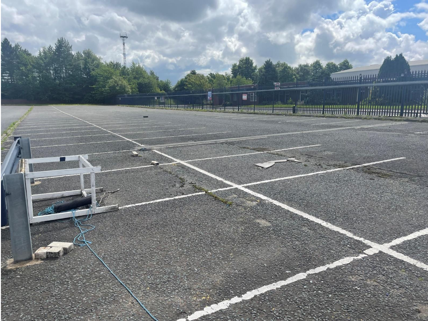
Photo 32: Car park in south eastern side of the site, looking south.
