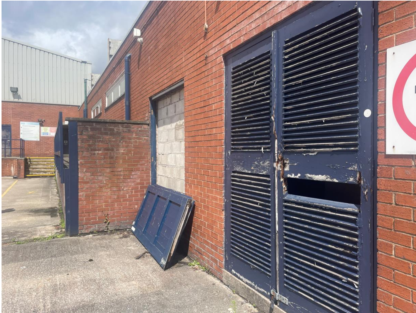
Photo 20: Southern end of the red brick building looking west. The doors to boiler house are to the right of the photo.
