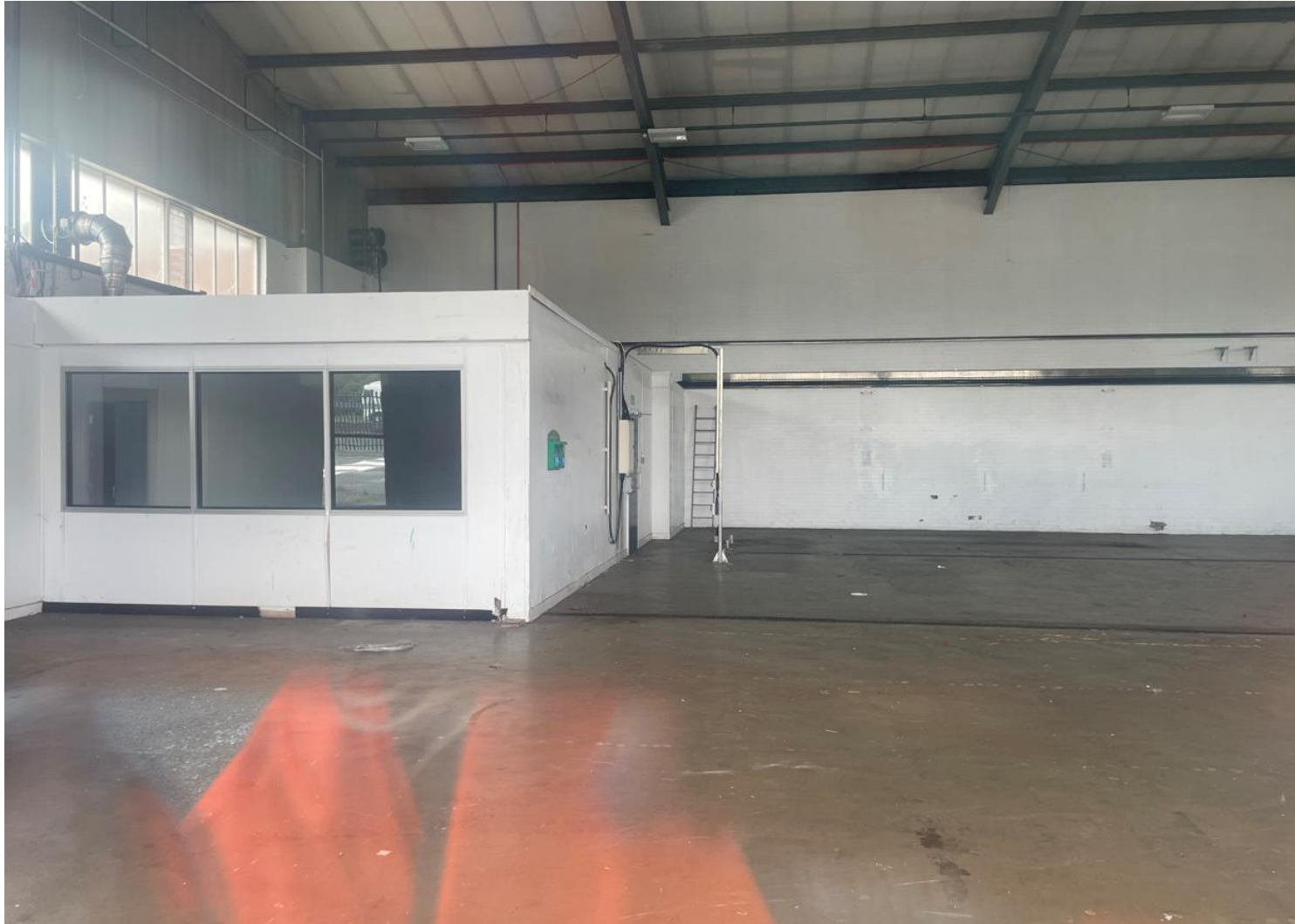
Photo 14: View through windows on eastern side of the building. Shows area to be empty.
