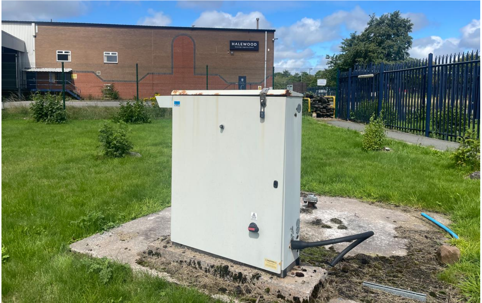
Photo 4: Possible electric box on concrete slab located in the north eastern part of the site.
