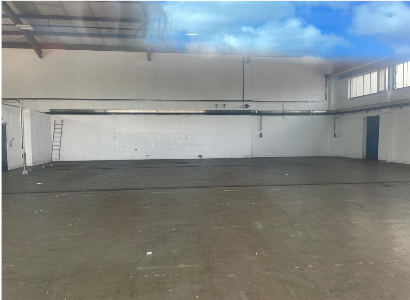
Photo 13: View through windows on eastern side of the building. Shows warehouse area to be empty.
