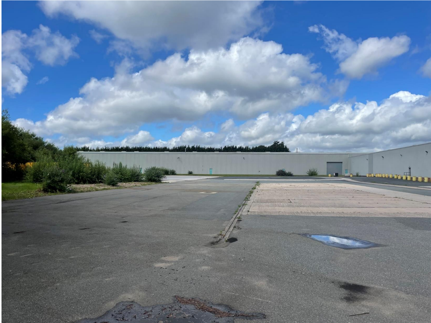
Photo 26: View looking north of the yard space area. Soft landscaping area in the left of the photo. Surface water drainage present in centre of hard surfacing.
