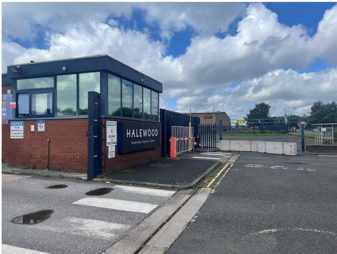
Photo 31: Access to the north eastern side of the site has been blocked off by concrete barriers.
