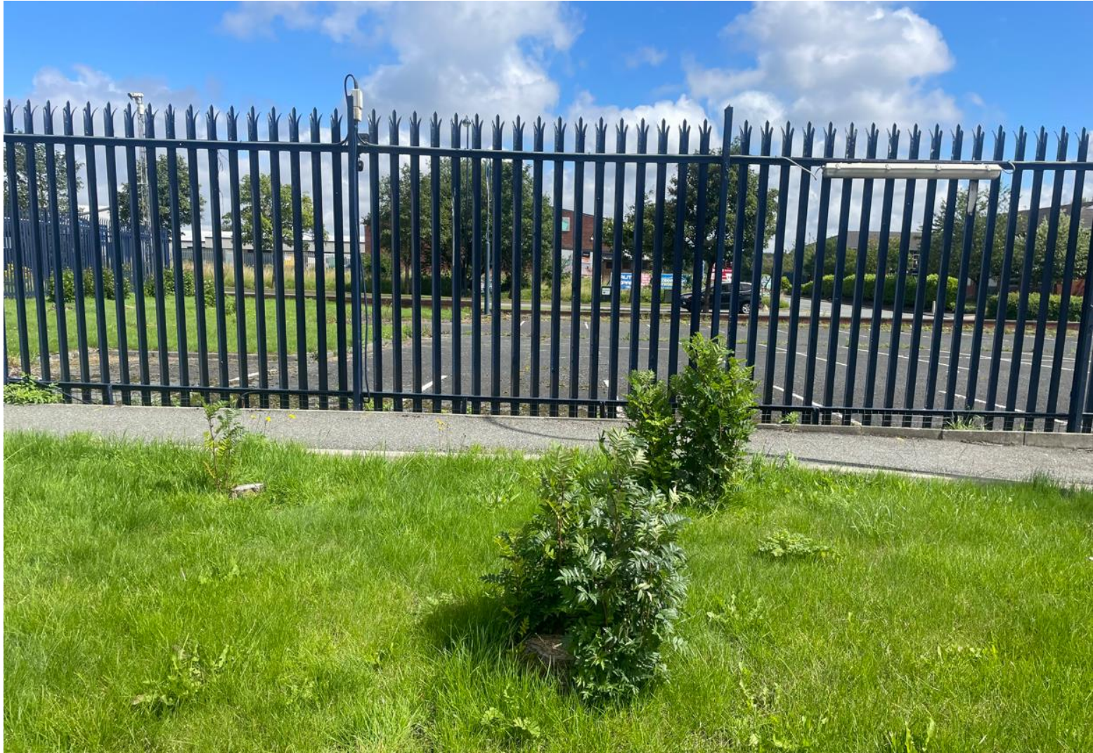
Photo 3: Palisade fencing creates barrier between onsite car park in eastern side of the site and access road visible in Photo 2. View is looking east.
