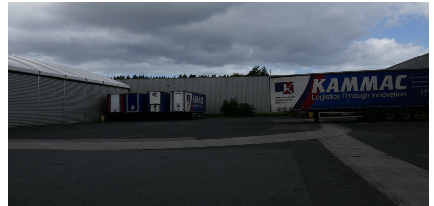
Junction of Block A and Block D within site which will be partly demolished.
