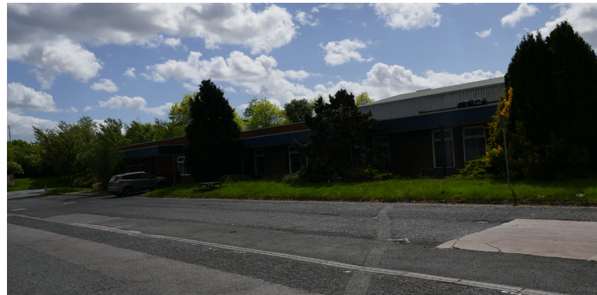
View of Block A single storey office extension to be demolished.
