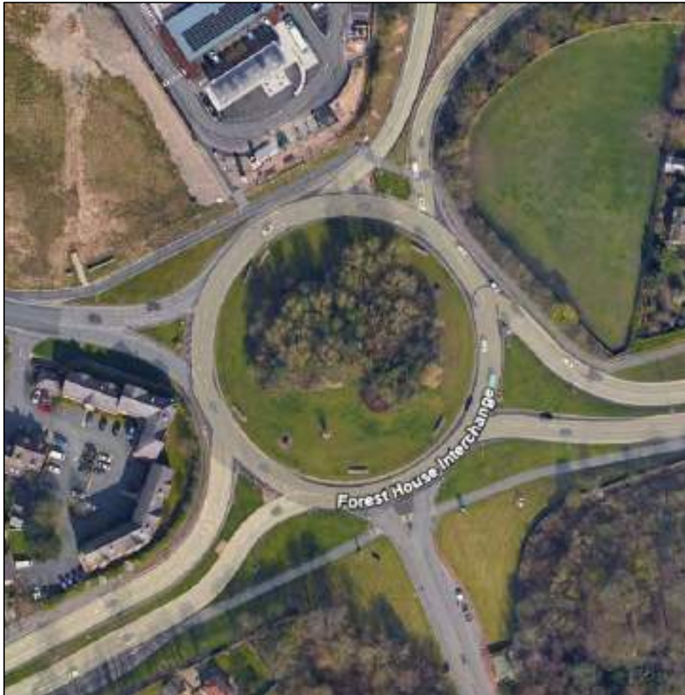
Figure 3.8: Forest House Interchange - M57 Junction 2 (Western Roundabout) (Source: Google Earth)
