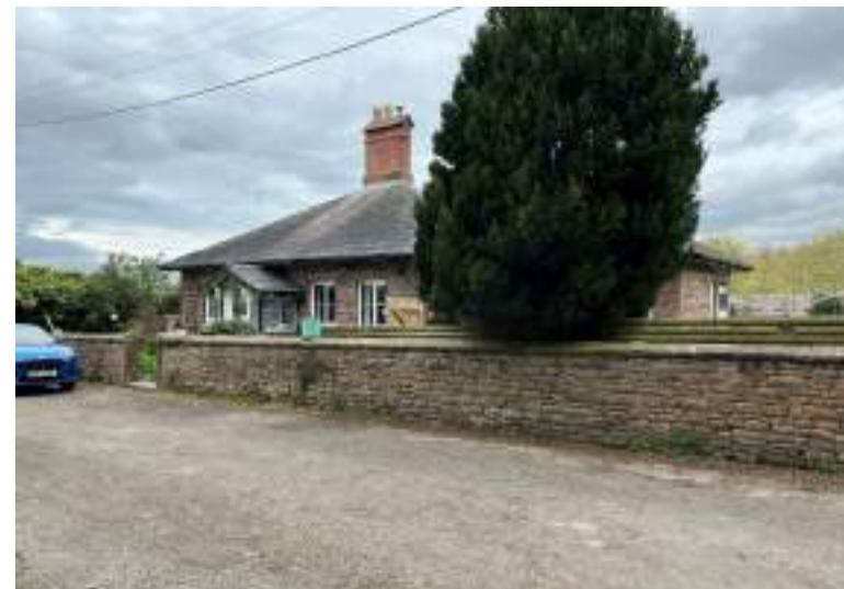
Plate 85: Home Farm Lodge, identified as likely curtilage listed to the Grade II* Listed Knowsley Hall.
