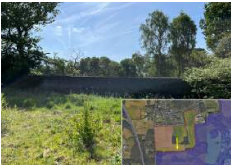
Plate 57: The open section on southern Site boundary.
