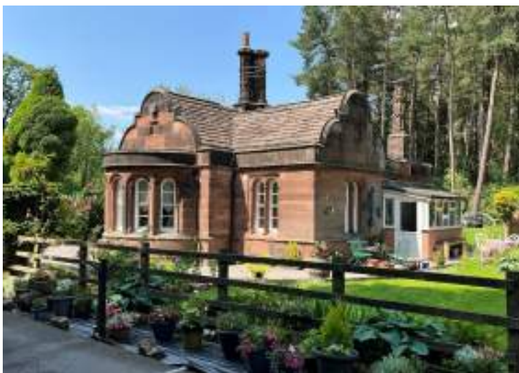
Plate 76: Croxteth Lodge, identified as curtilage listed to the Grade II* Listed Knowsley Hall.
