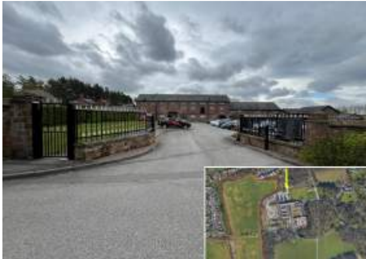
Plate 105: The principal access to Home Farm.
