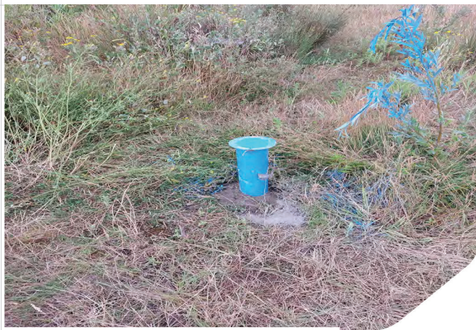
Photo 09: Standpipe of completed borehole WS07
