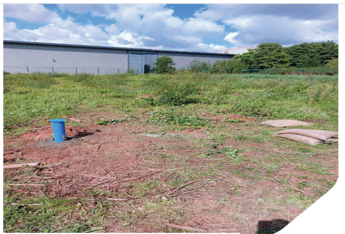
Photo 10: Standpipe of completed borehole CP02
