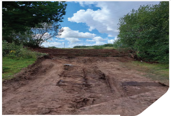
Photo 02: View of reinstated earth bund in Parcel 1 from the east
