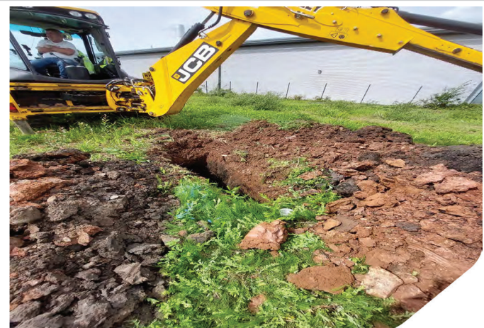
Photo 06: JCB 3CX excavating TP03 in Parcel 2
