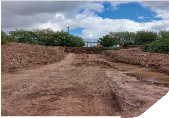
Photo 01: View of reinstated earth bund in Parcel 1 from the west
