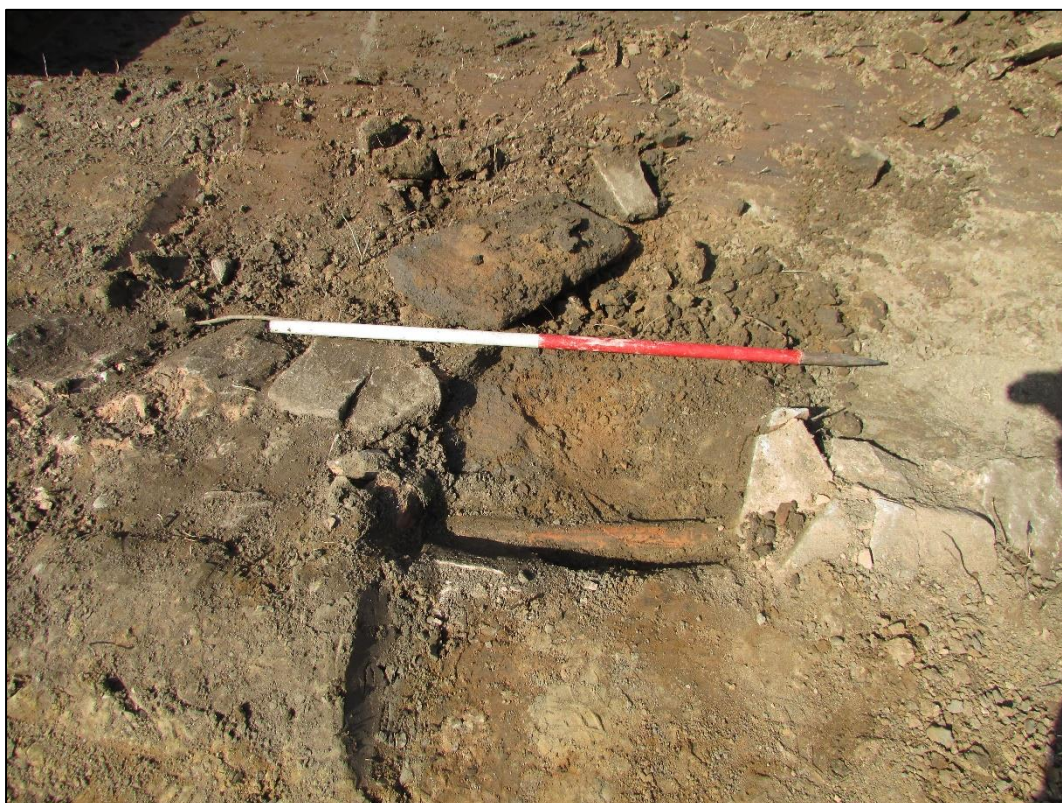
Plate 15: Ceramic drain (05)
