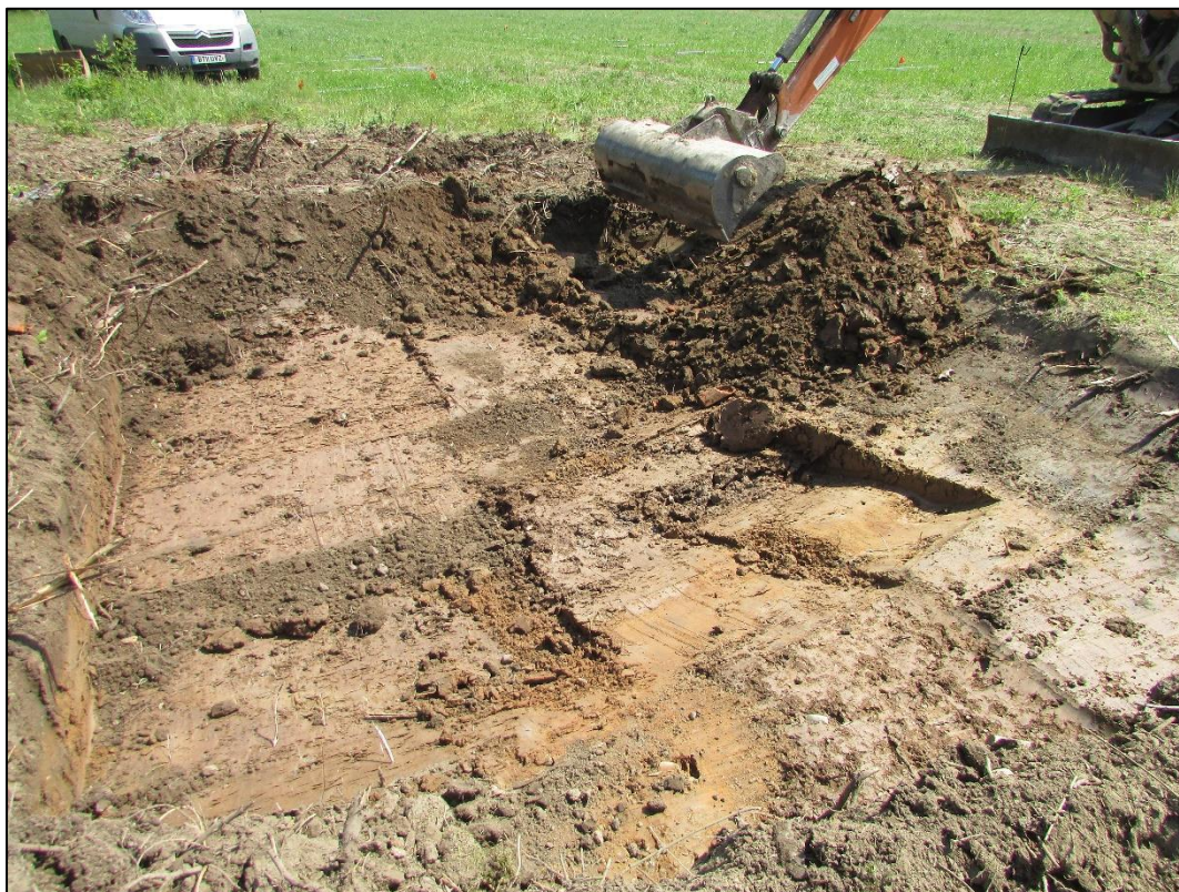
Plate 12: Working shot of trench 2 excavation
