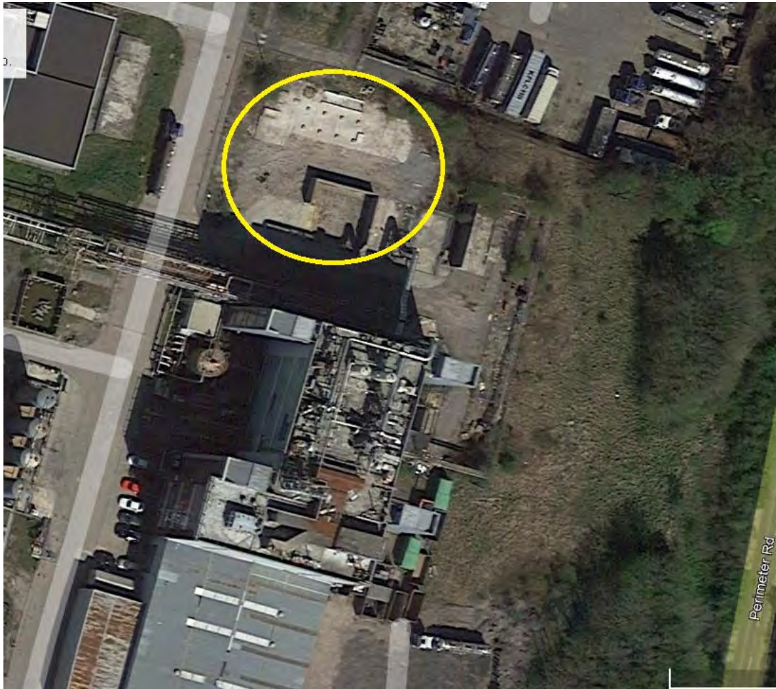
Figure 7.1 Plant, materials, and site compound
