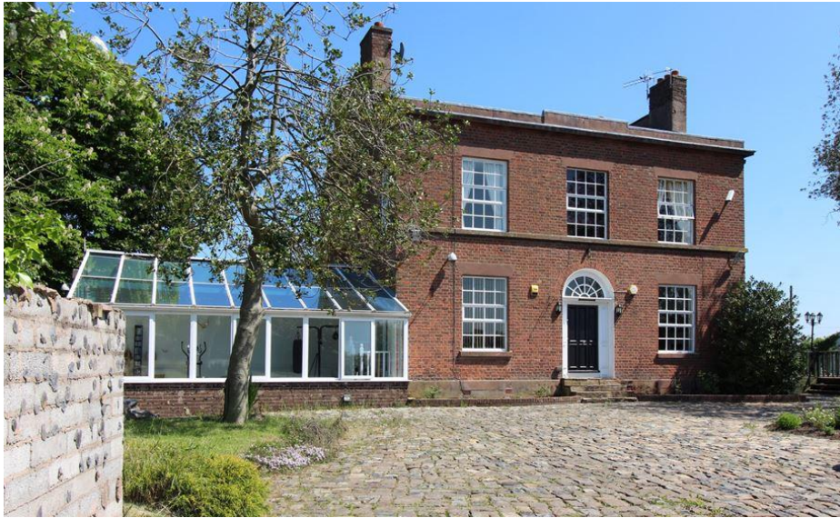
Figure 2: Image showing the front of the property
