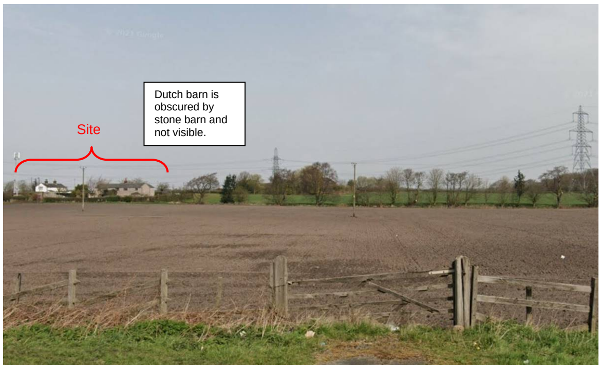
View 1: Looking north from East Lancashire Road. The existing buildings to be retained provide the dominant features. This view will remain unchanged.
