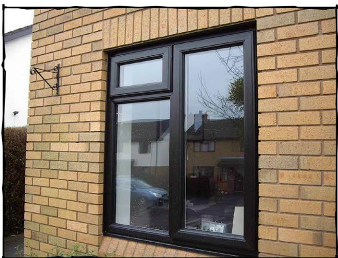
Black UPVC casement windows and doors
