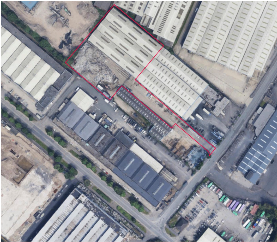
Fig 2. Aerial photo of the site prior to fire and subsequent demolition
