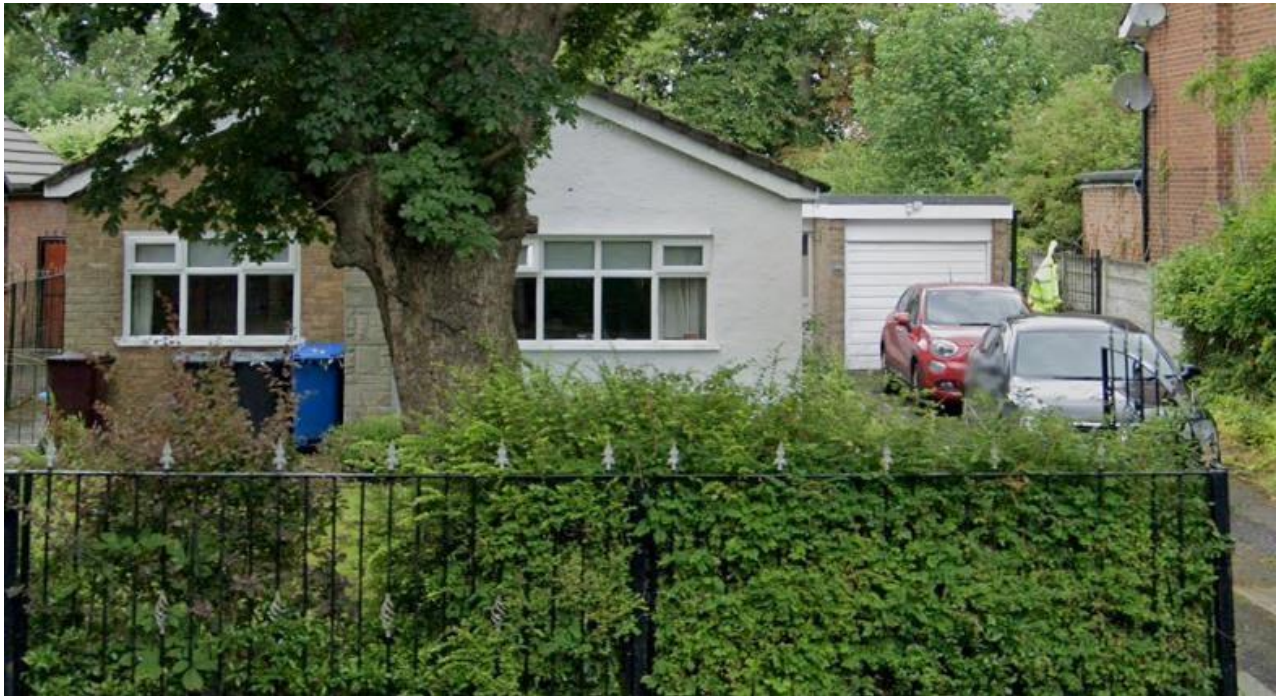
Photograph of existing front elevation
