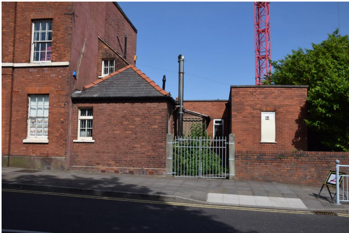
Figure 25: Church Street – outbuildings south of no 34 Cockpit House, from W (DSC_0463) in May 2020
