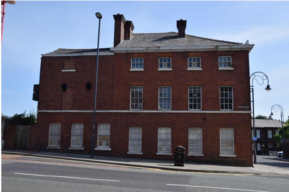
Figure 24: 34 Church Street (Cockpit House), from N (DSC_477)
