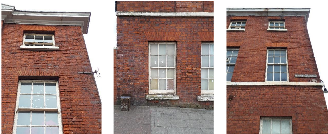
Figure 4: Instances of fabric repair required, some flat arches replaced, and displaced cornices.
