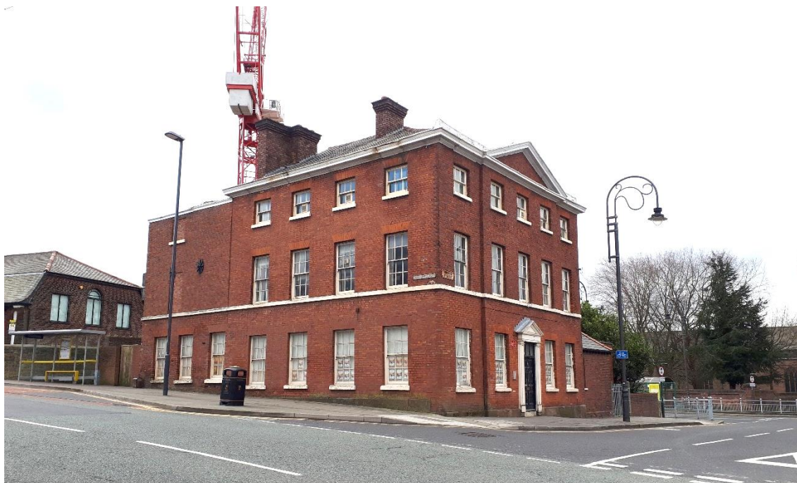
Figure 1: View of north and west elevations at intersection between High Street and Church Street
