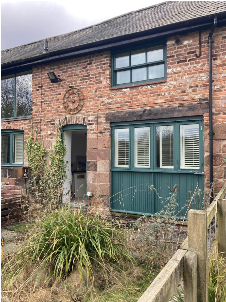
Fig.1 East facing elevation of Shippon 2 viewed from garden
