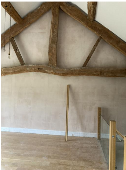
Fig.12 Roof truss at Party Wall. 1 st Floor Shippon 2
