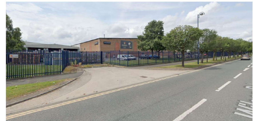
View B - View from Wilson Road towards existing site access SE of the site.
