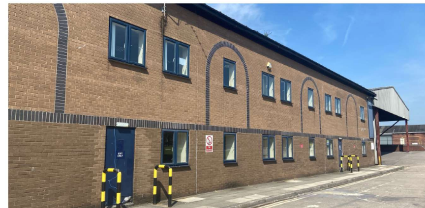
View C - View within the site toward the existing facade of Unit F.
