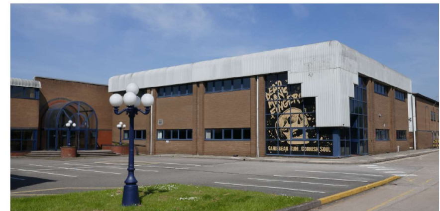
View D - View within site towards existing building to be demolished.
