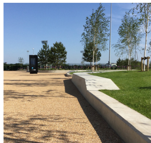
IN-SITU EXPOSED AGGREGATE AGAINST CONCRETE WALL
