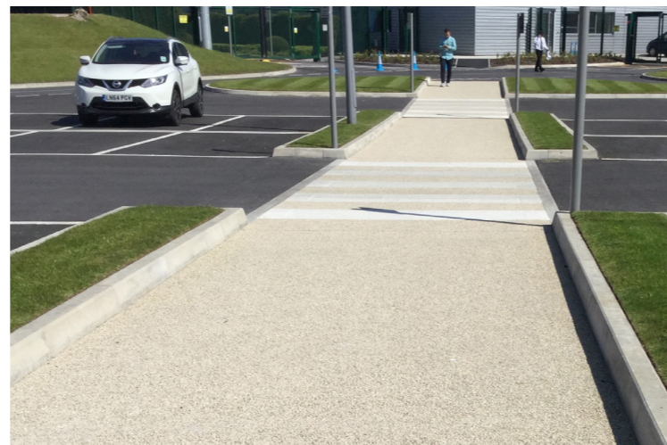
CONTRASTING COLOURS OF IN-SITU EXPOSED AGGREGATE CONCRETE
