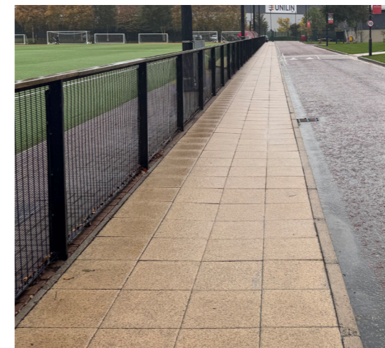
EXISTING SQUARE FORMAT CONCRETE PAVING
