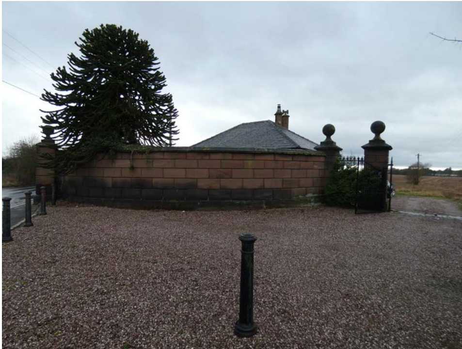
3.10 North East Lodge and Entrance Gates (Insalls)
