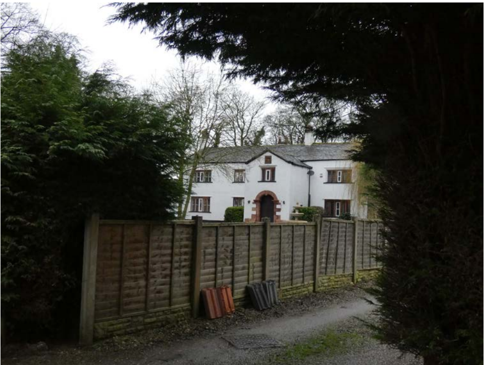
3.23 East boundary between Old Halsnead and Halsnead Villas (Insal)
