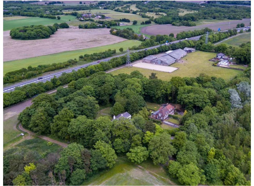
3.30 Aerial of Old Halsnead taken from 100m (Dragonflight Drones)
