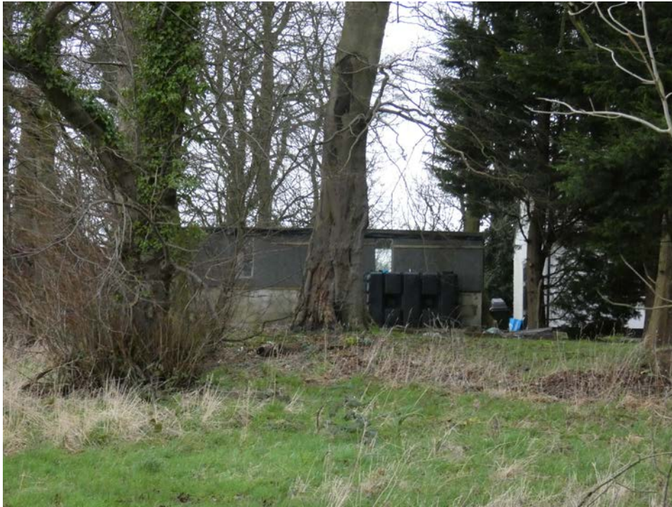
3.29 View of Outbuilding adjacent to Old Halsnead (Insall)
