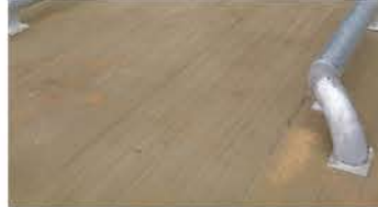
Concrete to yard areas and building circulation footpaths
