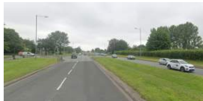
View on A506, Toward Fazakerley
