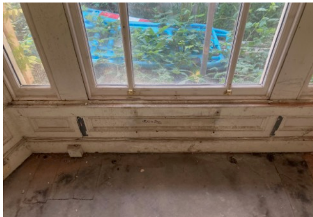
Fig.5 : Newly installed double-sliding sash windows with original outer frames / surrounds retained where present
