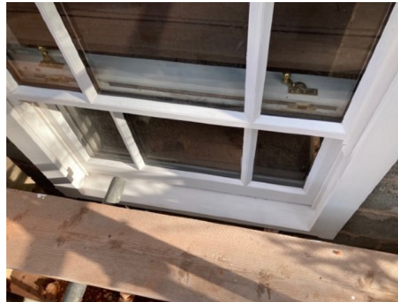
Fig.5 : Newly installed double-sliding sash windows with original outer frames / surrounds retained where present
