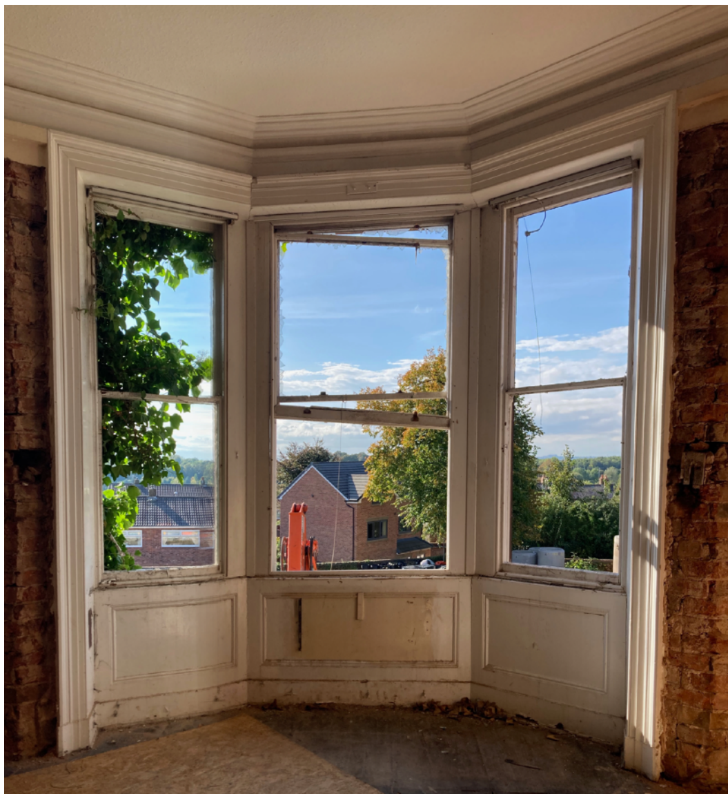
Fig. 3: Existing bay viewed from inside (windows W65, W66, W67)
