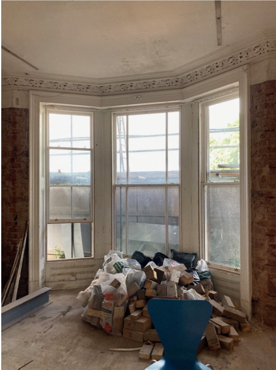
Fig.6 : Newly installed double-sliding sash windows with original outer frames / surrounds retained where present
