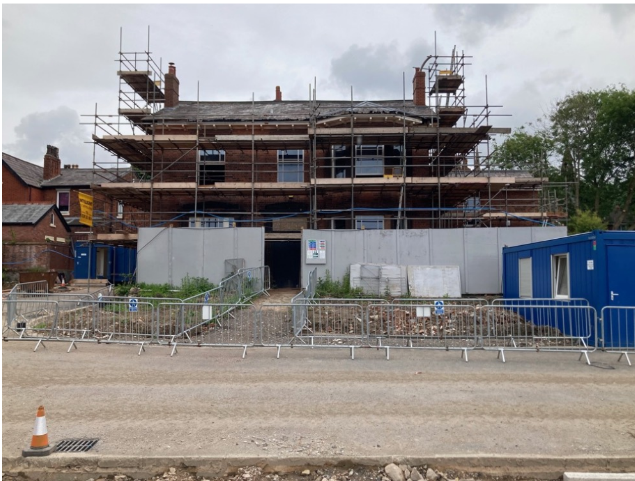
Fig. 7: Woodcroft front elevation showing newly installed double-sliding sash windows
