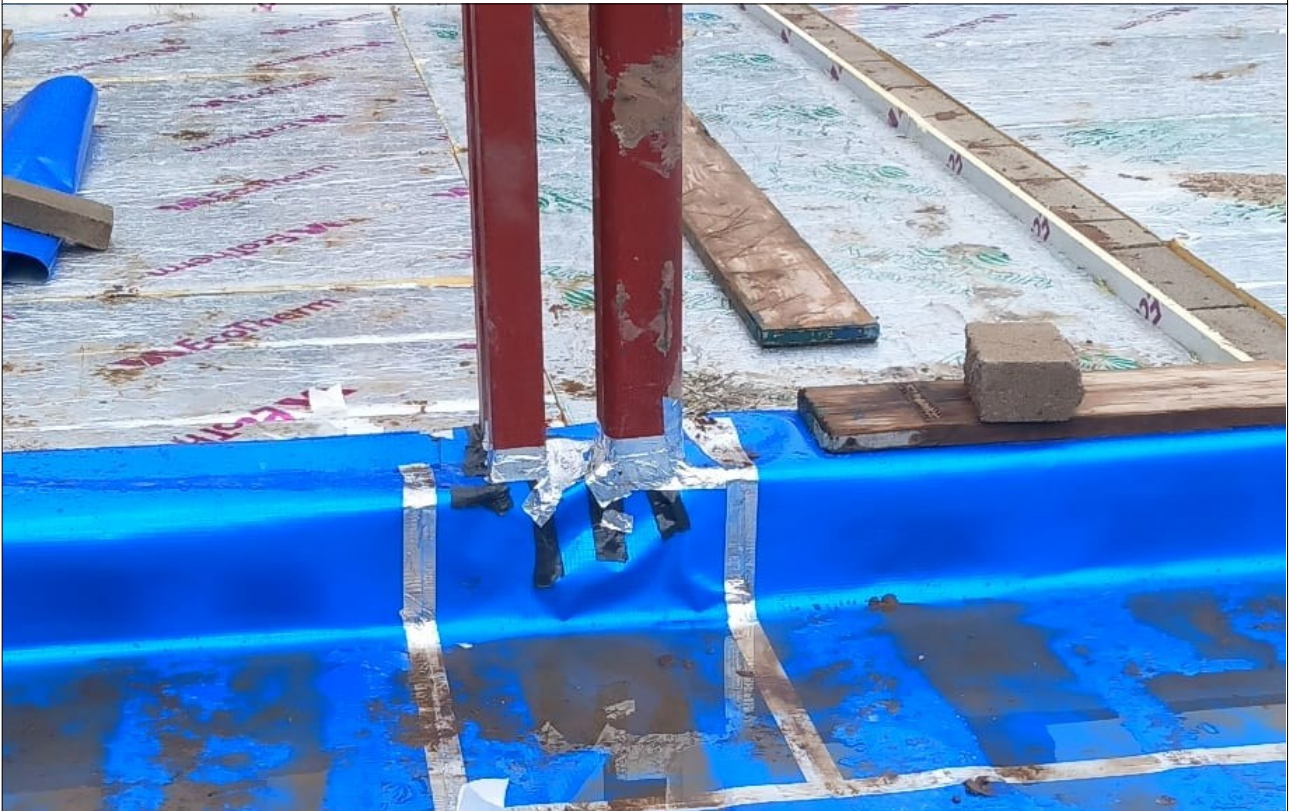
Plate 23: Plots 5, 6 & 7 gas membrane general condition.
