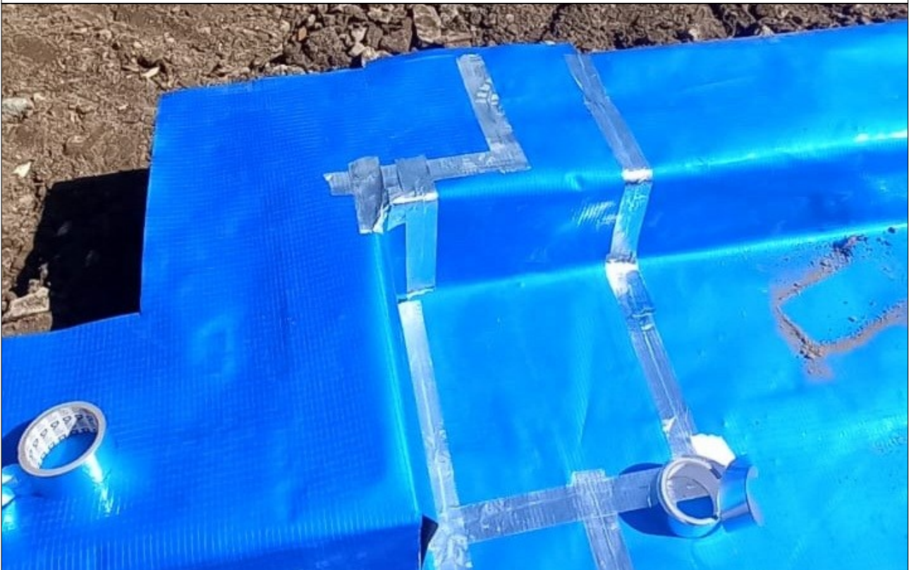
Plate 30: Plots 8 & 9 gas membrane general condition.
