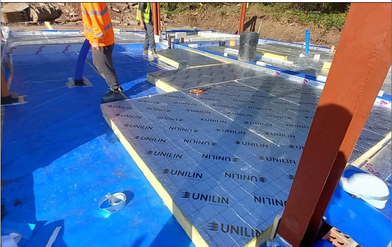
Plate 28: Plots 8 & 9 gas membrane general condition.
