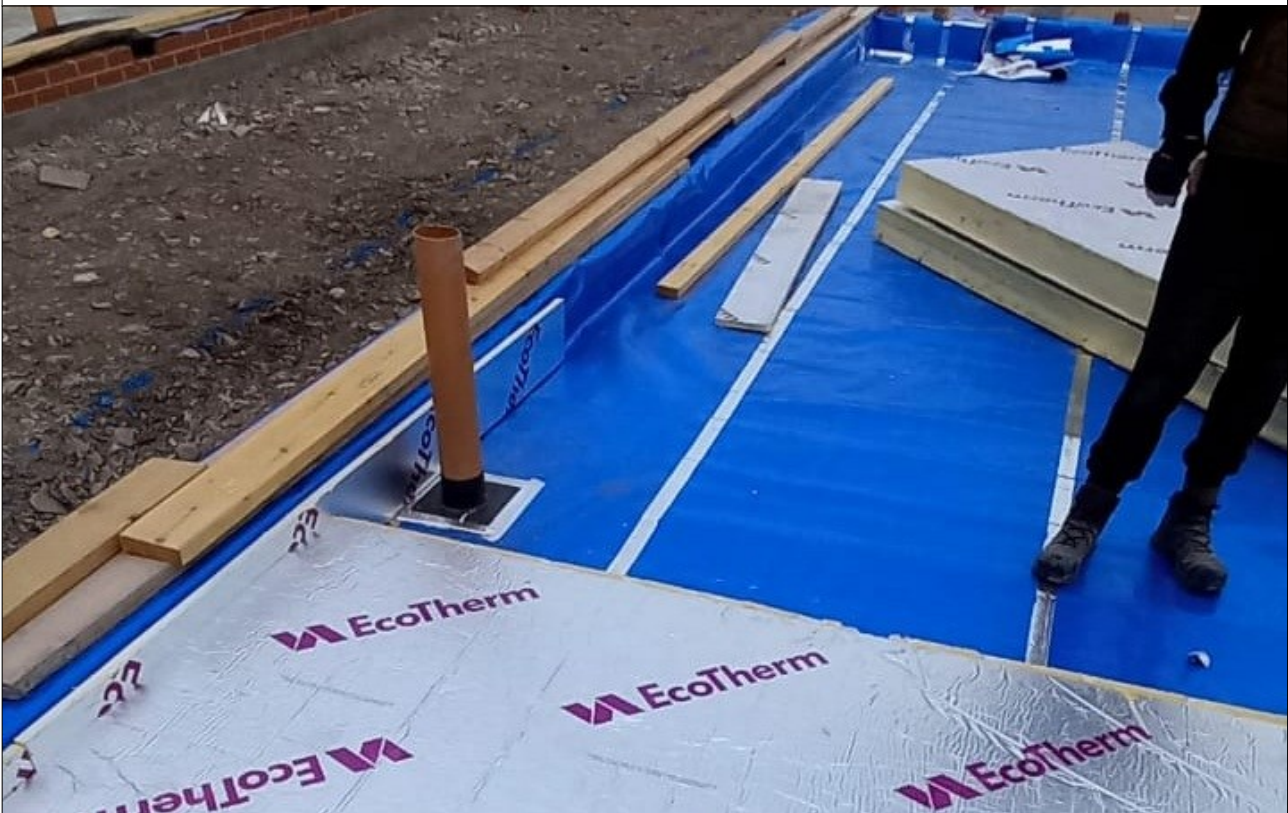
Plate 21: Plots 5, 6 & 7 gas membrane general condition.
