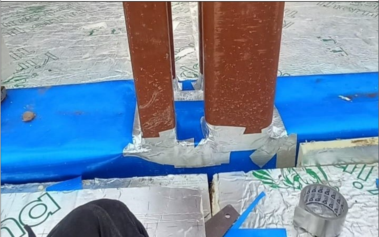
Plate 16: Plots 3 & 4 gas membrane general condition.
