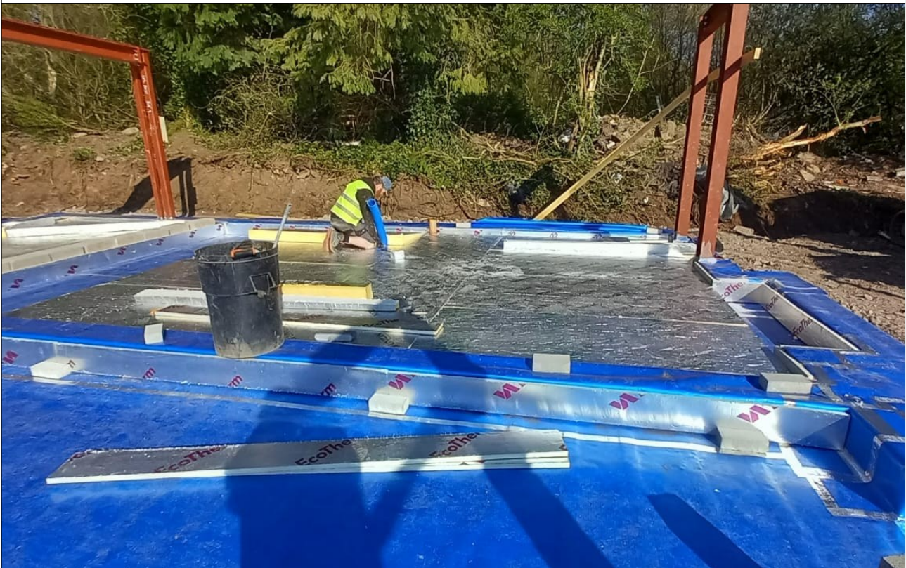
Plate 26: Plots 8 & 9 gas membrane general condition.
