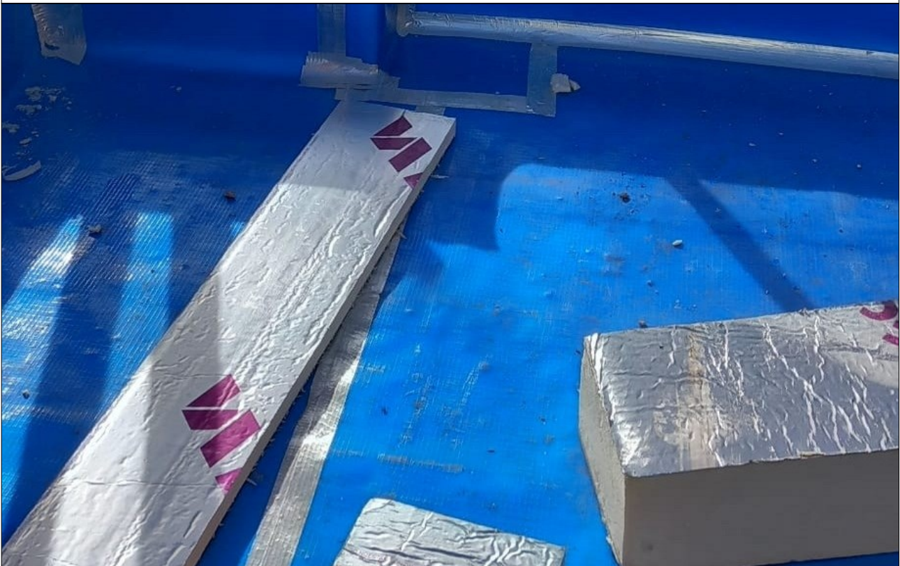
Plate 14: Plots 3 & 4 gas membrane general condition.
