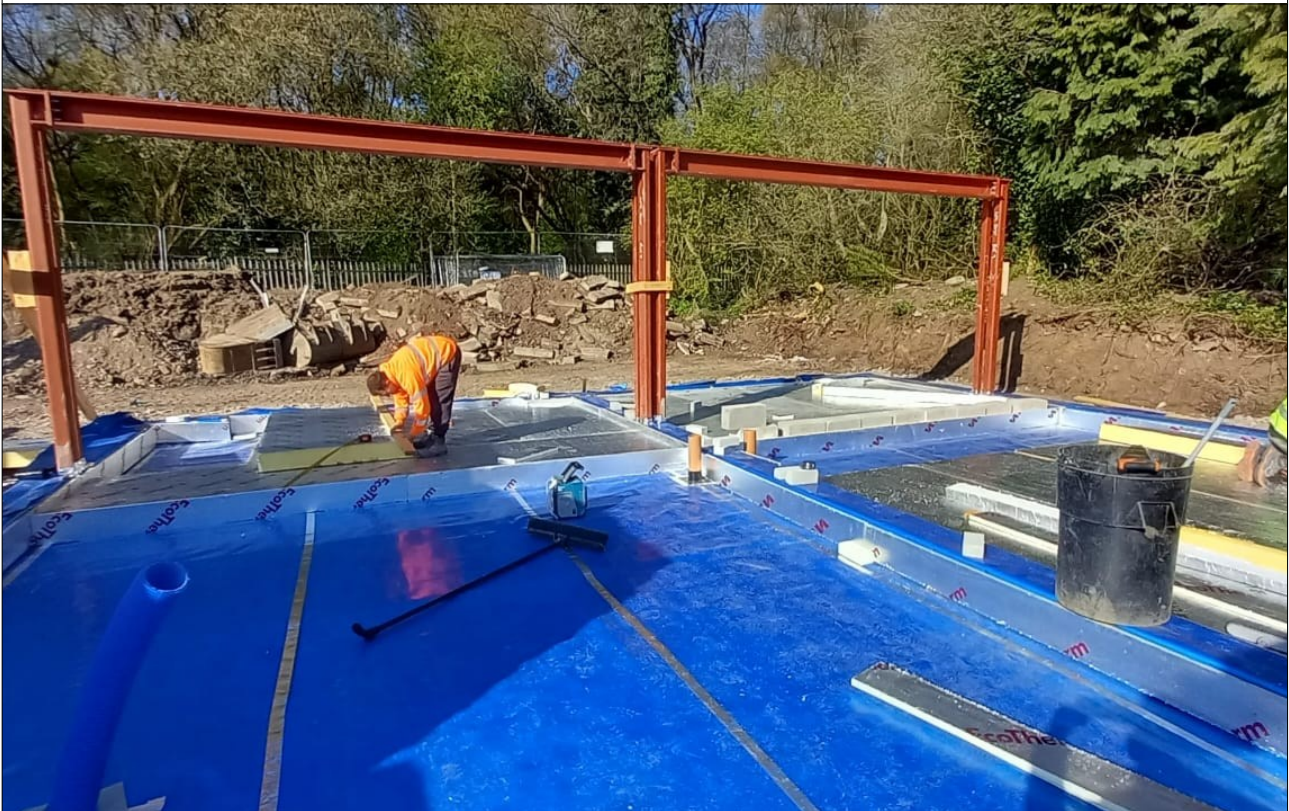
Plate 25: Plots 8 & 9 gas membrane general condition.
