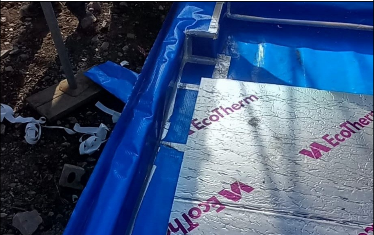
Plate 8: Plots 1 & 2 gas membrane general condition.
