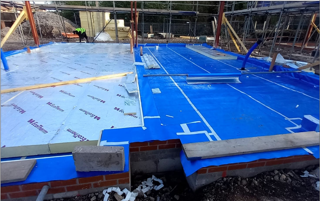
Plate 1: Plots 1 & 2 gas membrane general condition.
