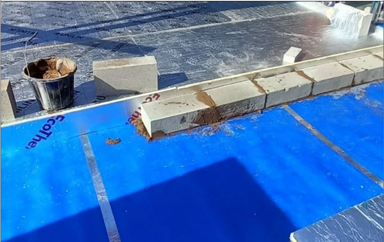
Plate 29: Plots 8 & 9 gas membrane general condition.
