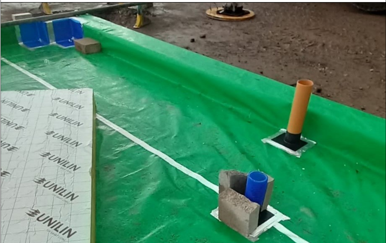
Plate 22: Plots 5, 6 & 7 gas membrane general condition.
