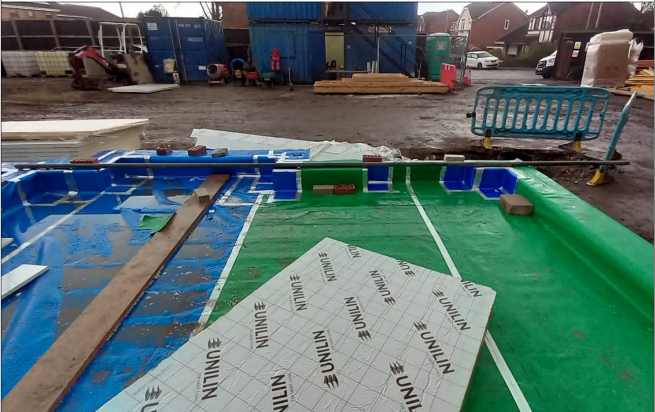
Plate 17: Plots 5, 6 & 7 gas membrane general condition.
