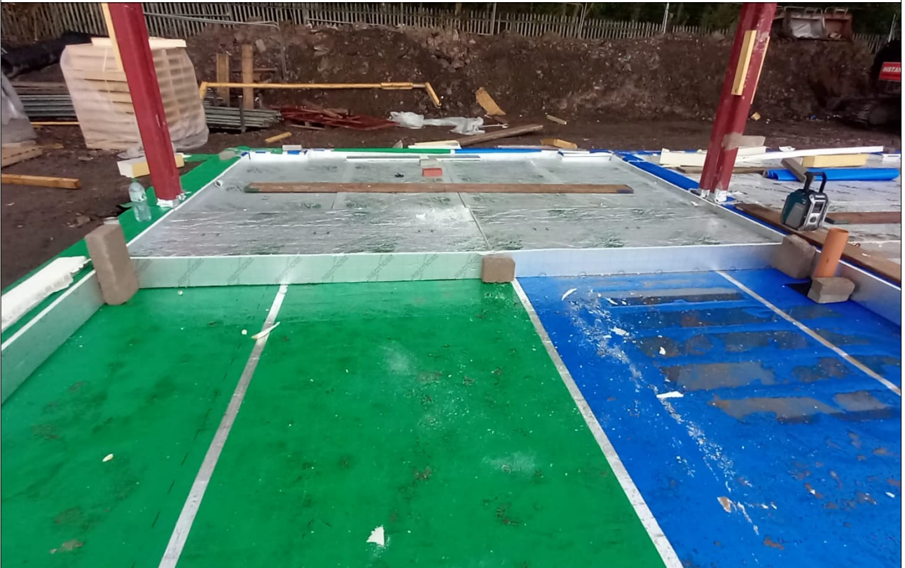
Plate 19: Plots 5, 6 & 7 gas membrane general condition.
