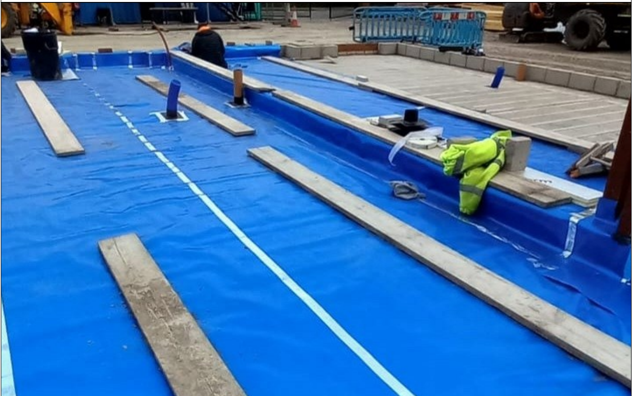
Plate 18: Plots 5, 6 & 7 gas membrane general condition.
