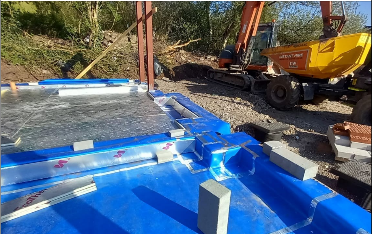
Plate 27: Plots 8 & 9 gas membrane general condition.
