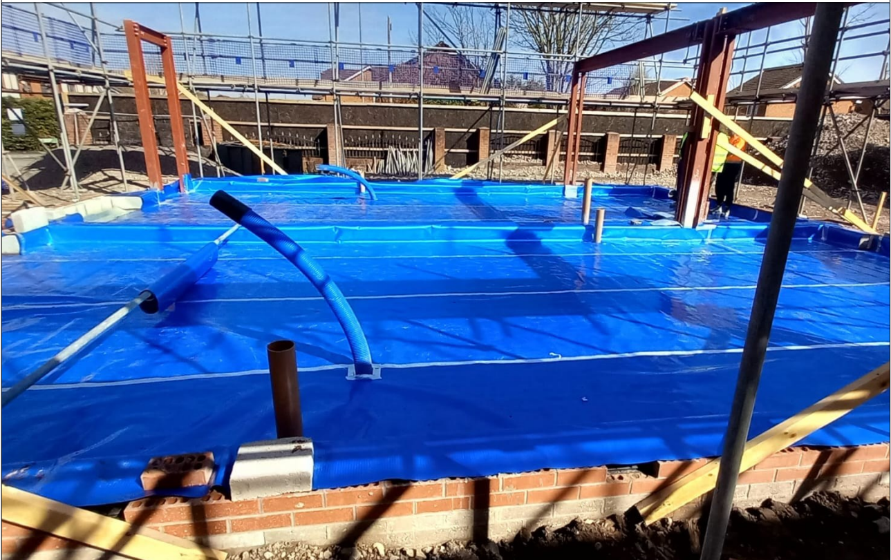
Plate 3: Plots 1 & 2 gas membrane general condition.
