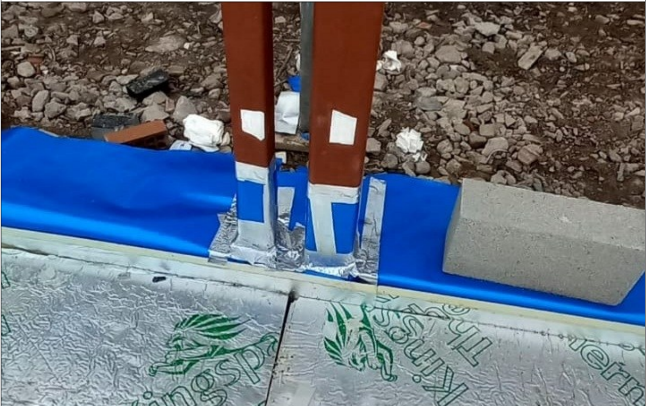
Plate 15: Plots 3 & 4 gas membrane general condition.
