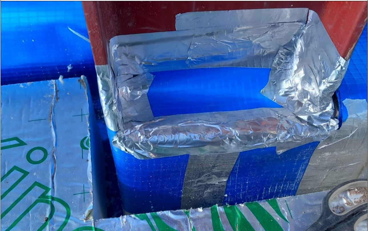
Plate 11: Plots 3 & 4 gas membrane general condition.
