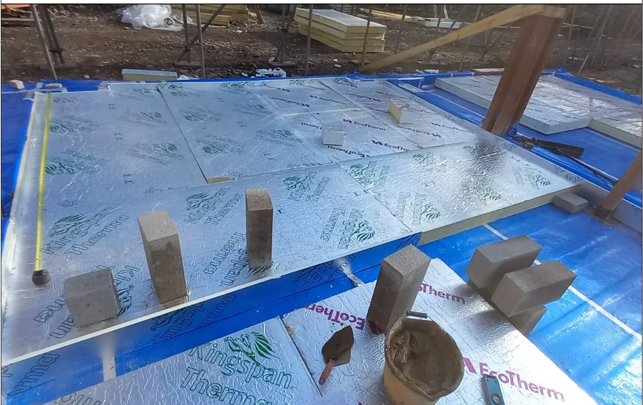
Plate 2: Plots 1 & 2 gas membrane general condition.
