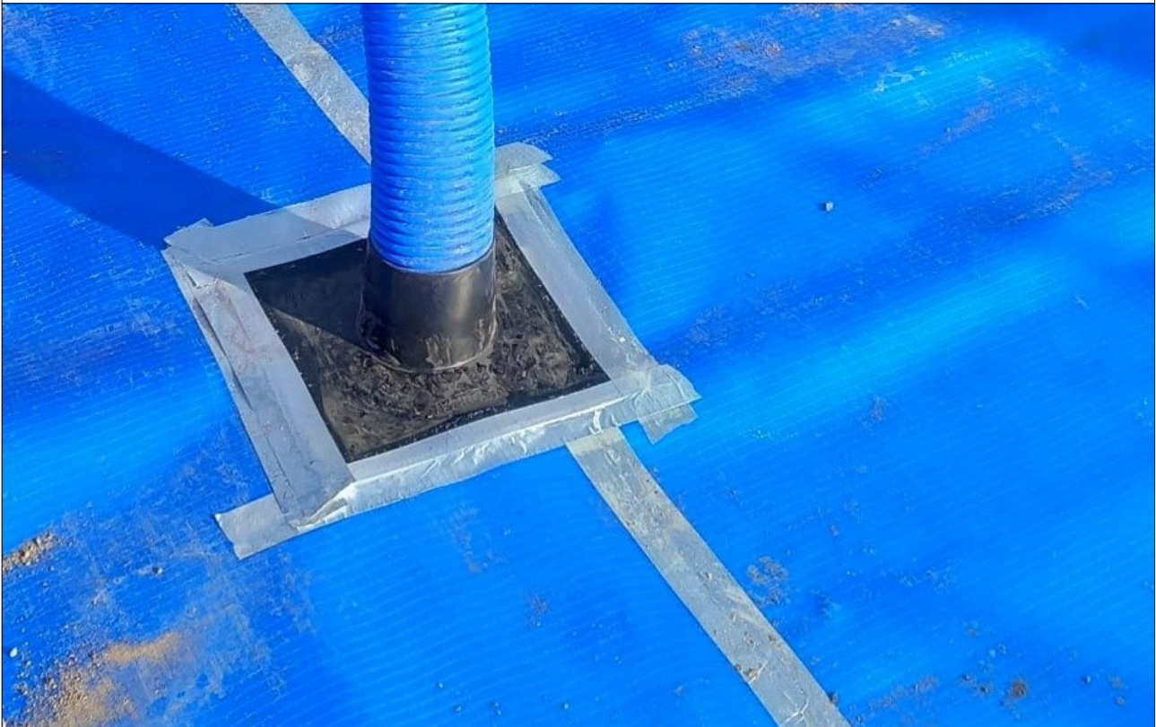
Plate 5: Plots 1 & 2 gas membrane general condition.
