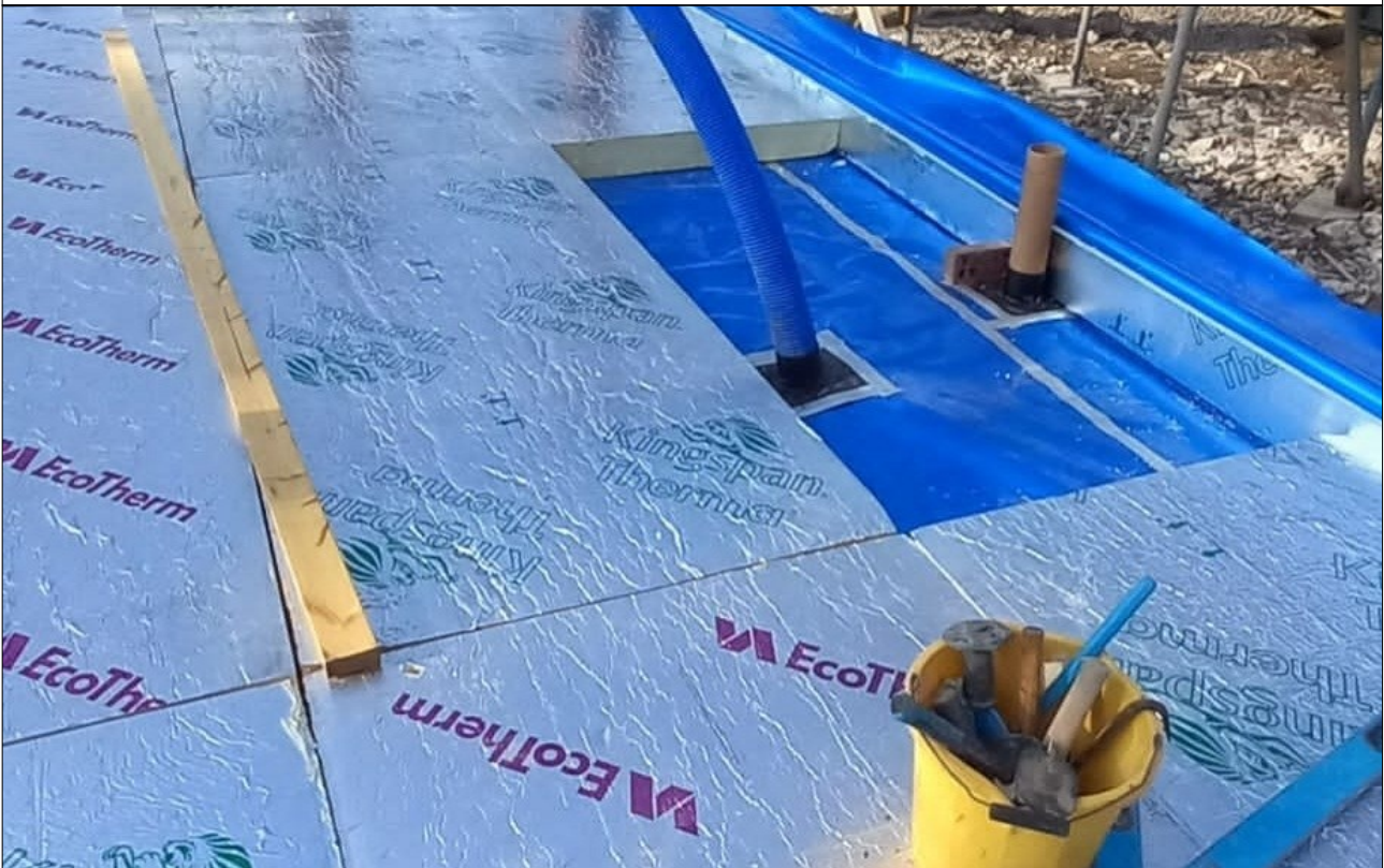
Plate 6: Plots 1 & 2 gas membrane general condition.
