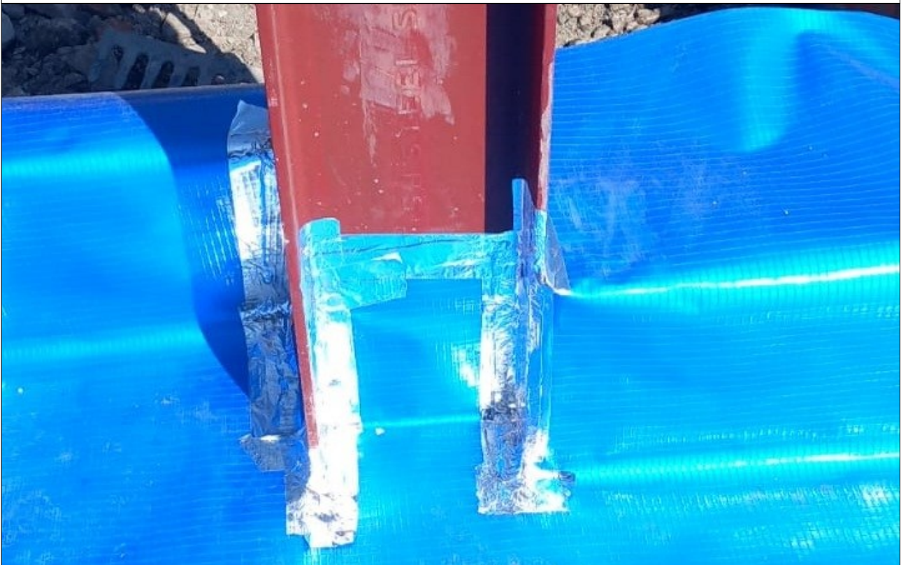
Plate 32: Plots 8 & 9 gas membrane general condition.
