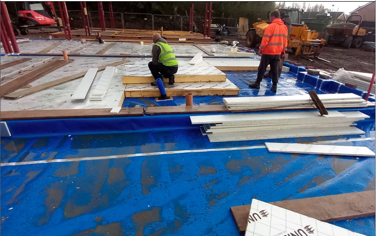
Plate 20: Plots 5, 6 & 7 gas membrane general condition.
