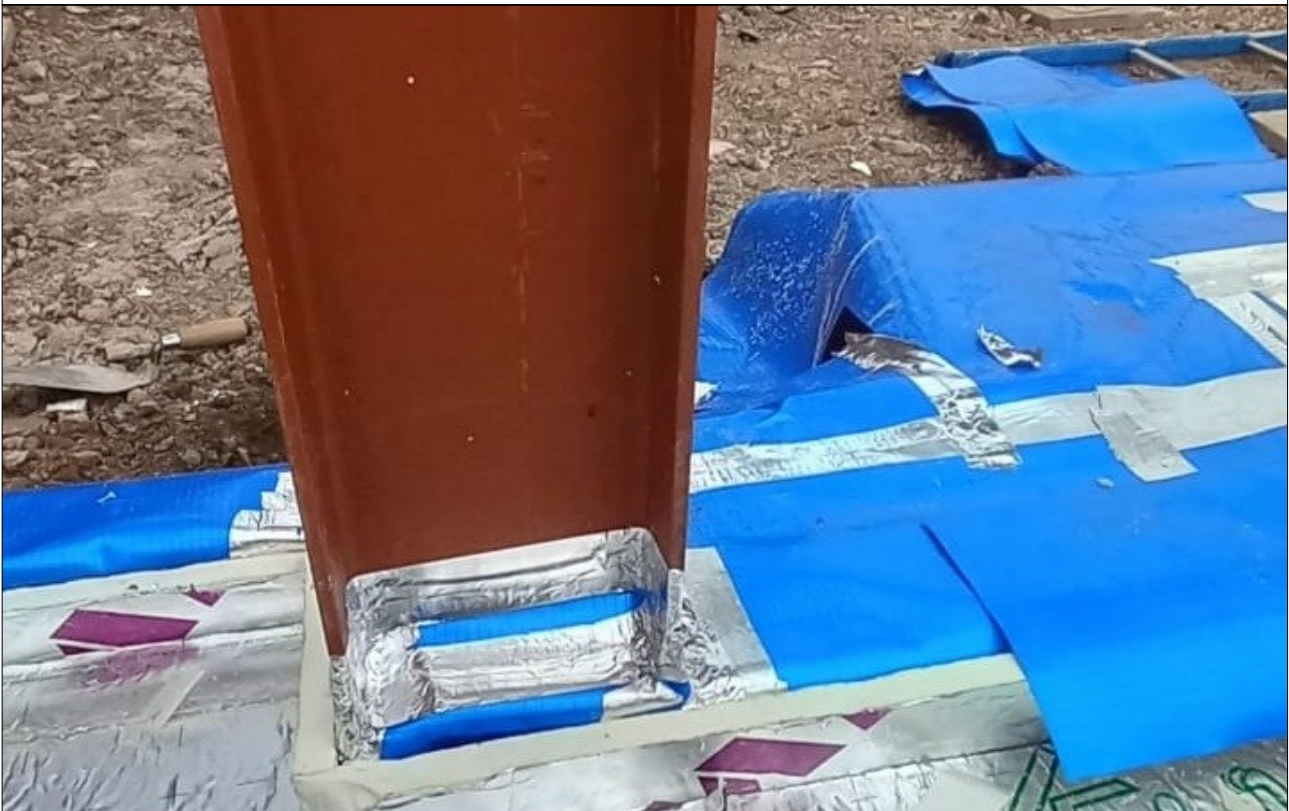
Plate 12: Plots 3 & 4 gas membrane general condition.
