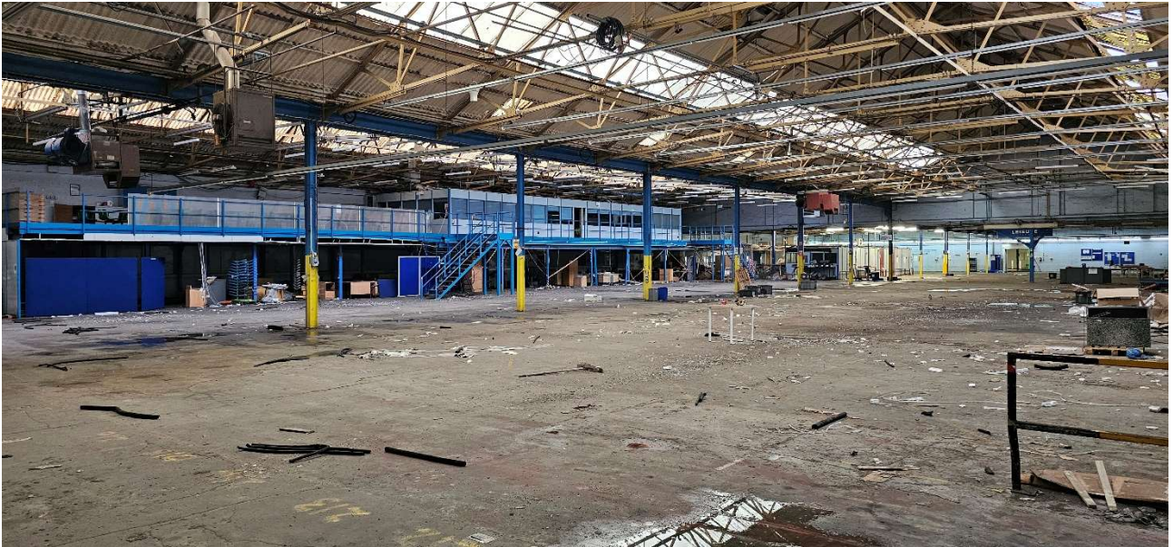
Image1F(1) – Interior of Building 1F looking west
