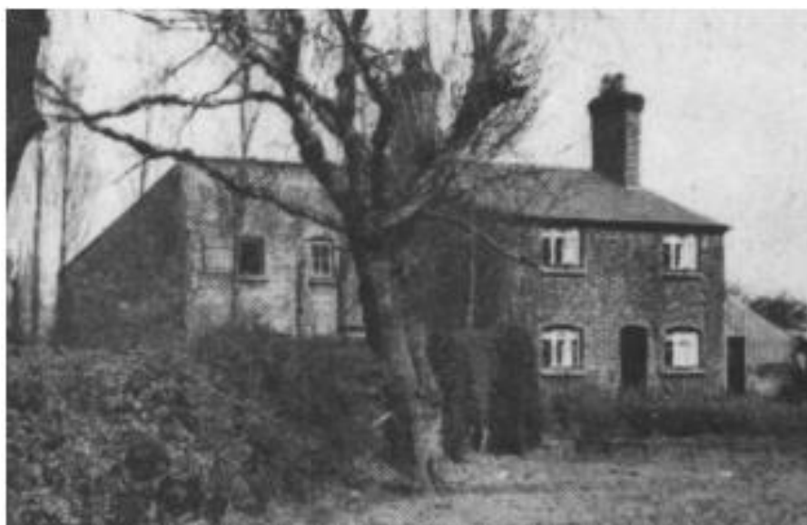
Figure 2 Extract from photograph dated 1926 showing Alderley from the South
