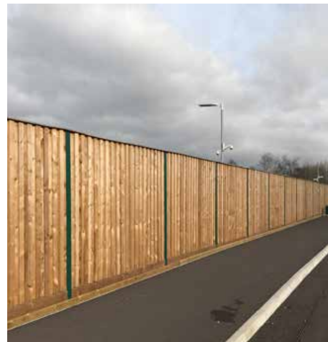
Typical Acoustic Fence
