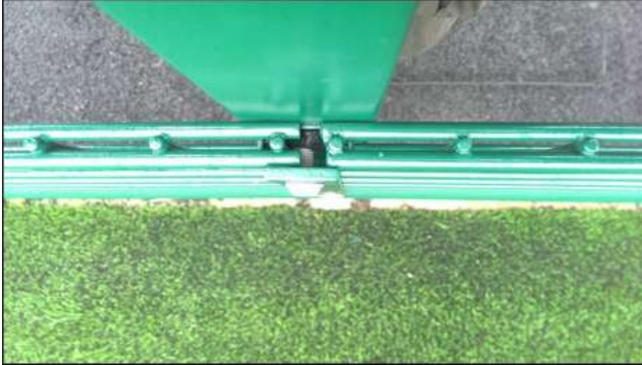
Figure 9: Image showing neoprene isolators
