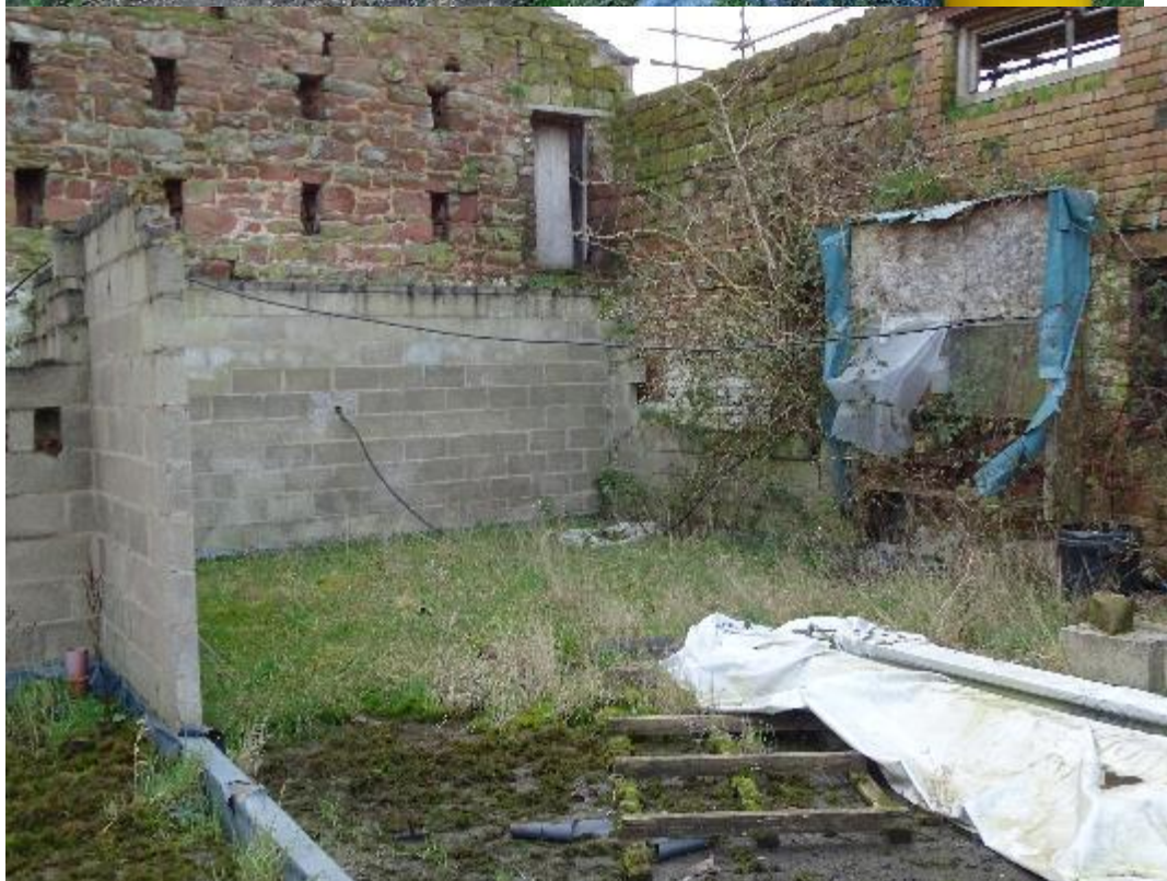
Single storey brick barn to rear of farmhouse
