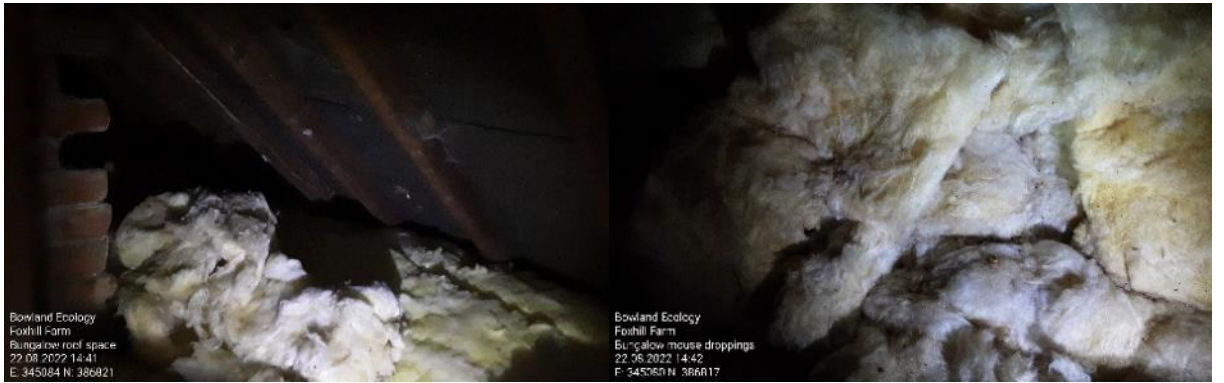
Plates 27 and 28: Loft voids (crawl space around upper rooms)
