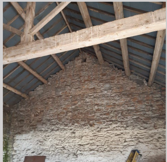
Photograph 4: Stone Barn A roof cavities
