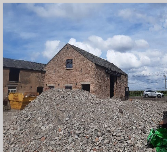
Photograph 22: Site construction material in courtyard.
