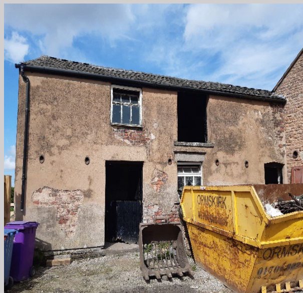
Photograph 9: Stone Barn B (eastern aspect)
