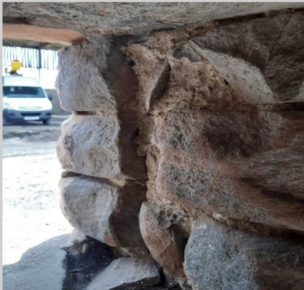
Photograph 3: Stone Barn A cavity wall view in window frame
