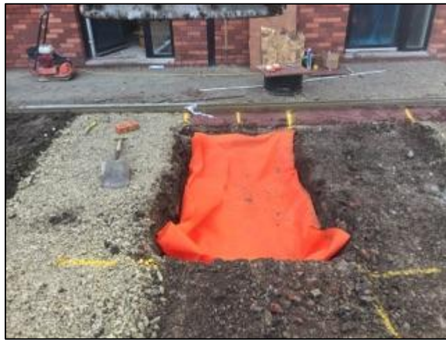
Figure 1: First, the gardens are dug out to 600mm below FFL and lined with a hi-viz geotextile marker:
