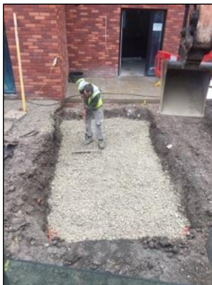
Figure 2: The geotextile is overlain by a 150mm clean stone break layer.
