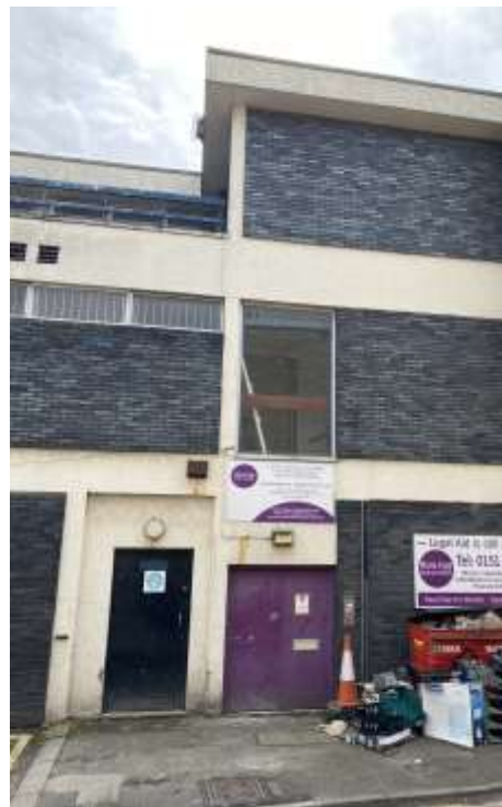
THE GROUND FLOOR FRONT ENTRANCE
