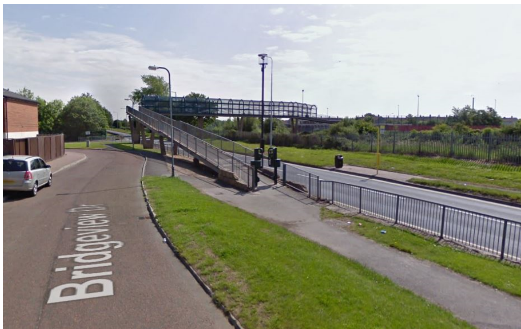
Figure 8: Pedestrian bridge located to the east of the development site
