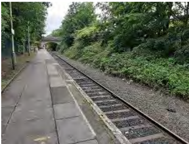
Photograph 11. Northern platform of Kirkby (TN15), with bankside vegetation opposite including Japanese knotweed at base of bare ground for substation (TN13).
