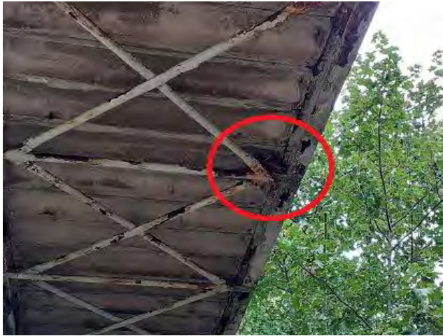
Photograph 19. Millbrook Bridge with gap present above arch ring.
