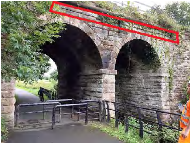
Photograph 19. Millbrook Bridge with gap present above arch ring.
