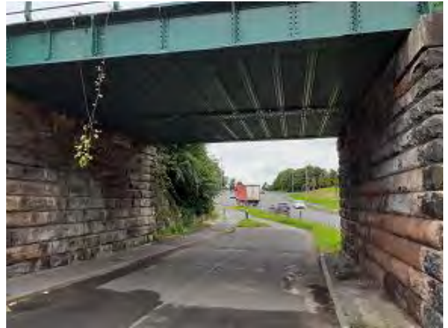
Photograph 20. Gap in arch of Millbrook Bridge near northern elevation, above footpath.
