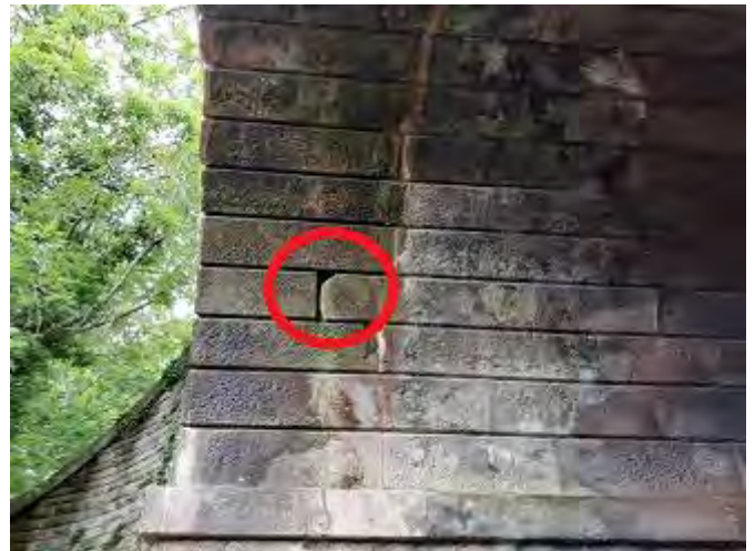
Photograph 20. Gap in arch of Millbrook Bridge near northern elevation, above footpath.
