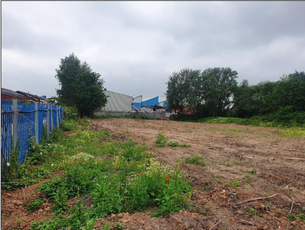
P1: Entire site (looking towards SW)
