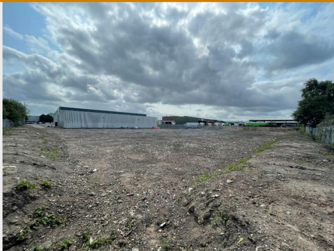
Photograph 1: Overview of the site and building B1 located near the centre of the site.
