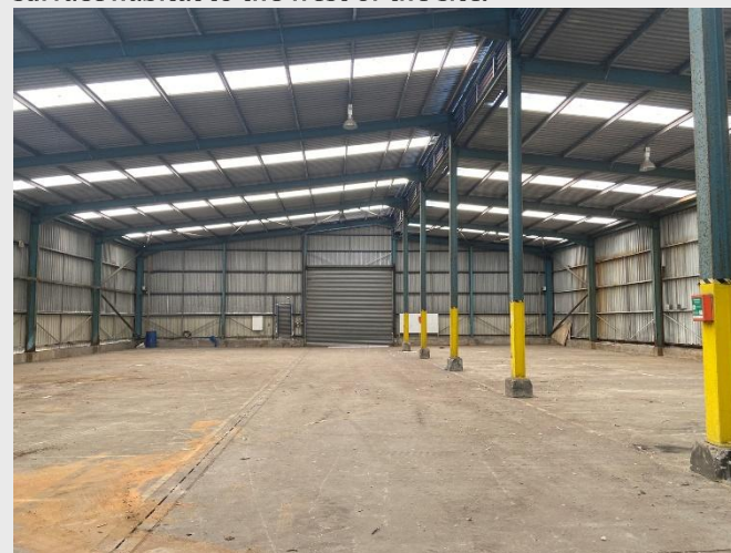
Photograph 4: Internal structure of B1 displaying internal artificial light and negligible roosting potential.
