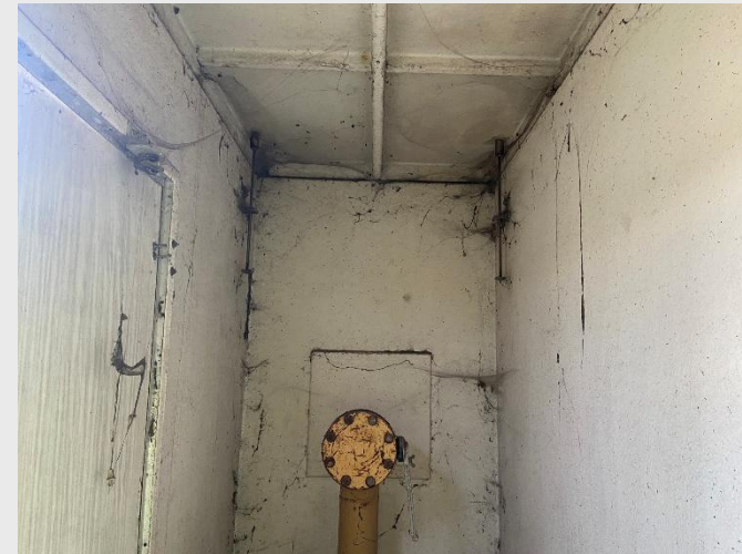
Photograph 6: Internal space of B2 showing lack of potential roosting features.
